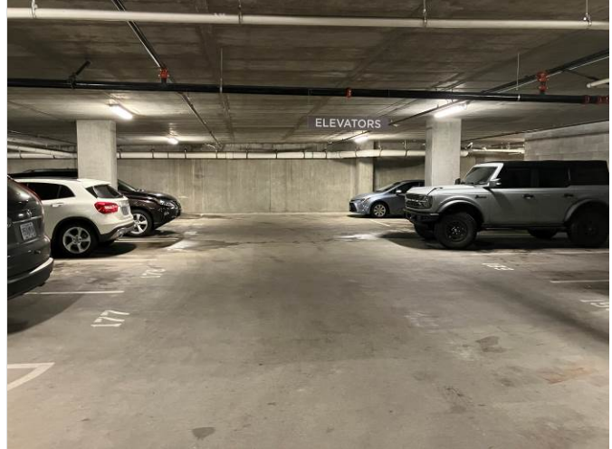
14. Parking garage/foundation view.
