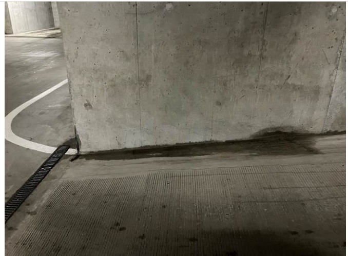
16. Parking garage ramp.
