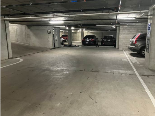
13. Parking garage/foundation view.
