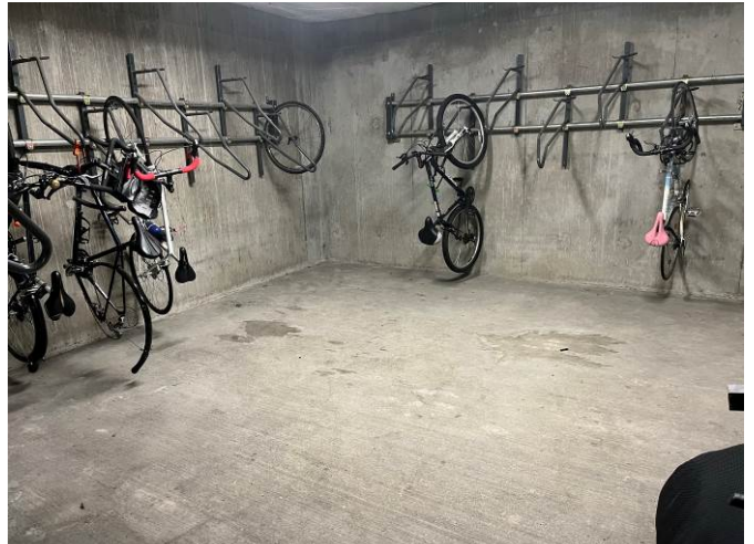
2. Parking garage/building foundation view A
