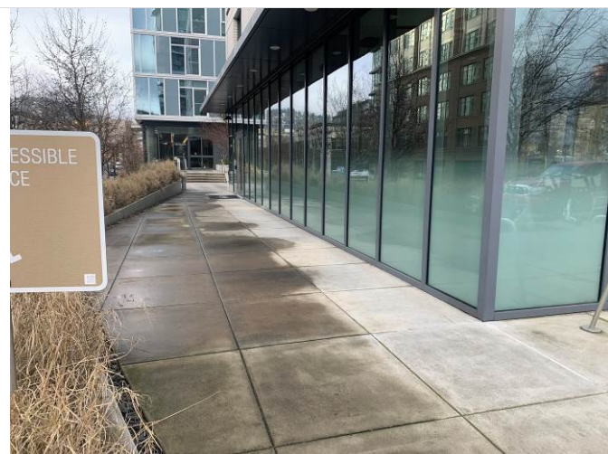
17. Hardscape along NW Overton St
