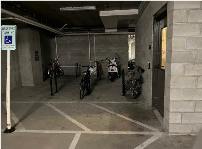
1. Bike Storage Area #1 in subterranean parking garage
