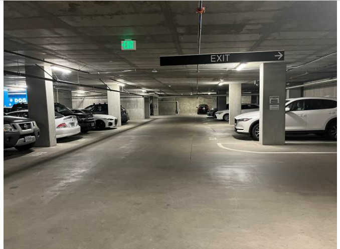
8. Parking garage/building foundation view D
