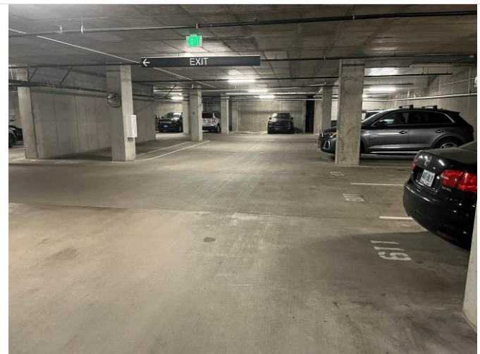
6. Parking garage/building foundation view C
