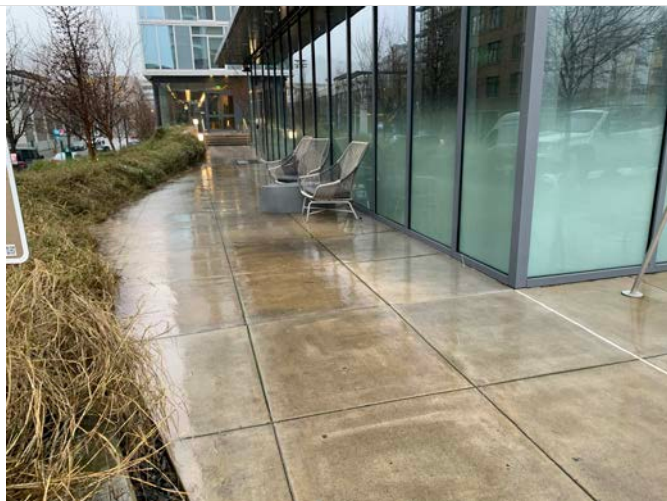
17. Hardscape along NW Overton St.
