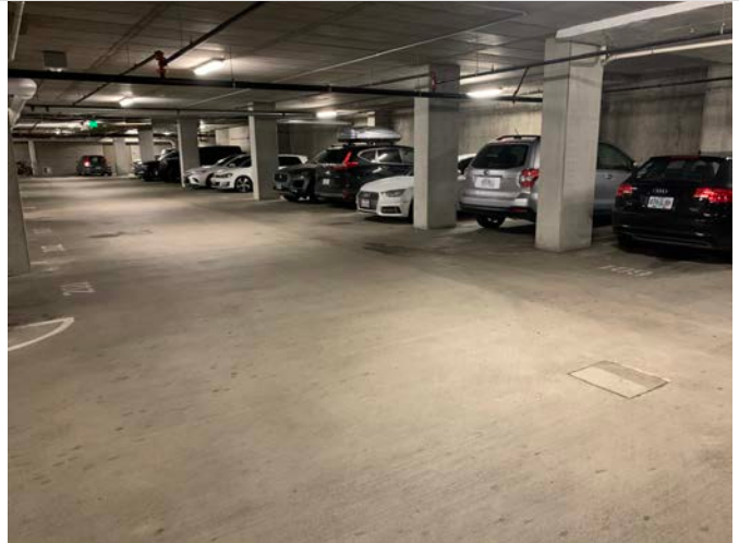
8. Parking garage/building foundation view D
