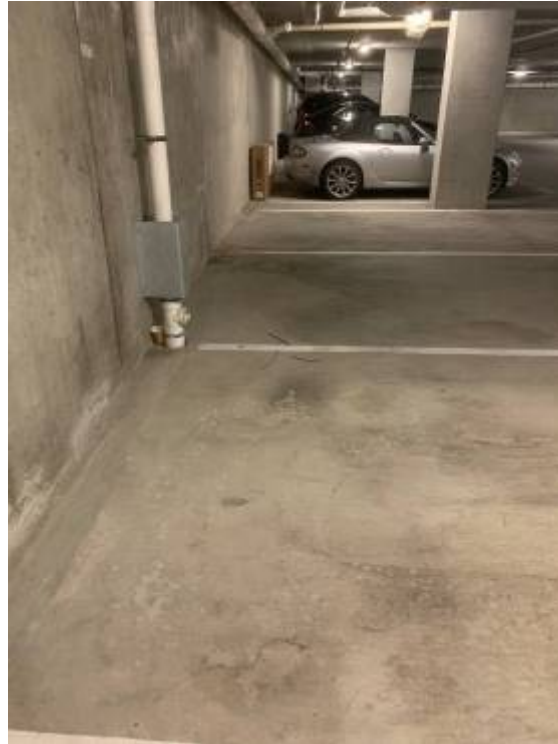
Photograph 1: Parking Garage Slab/Foundation A
