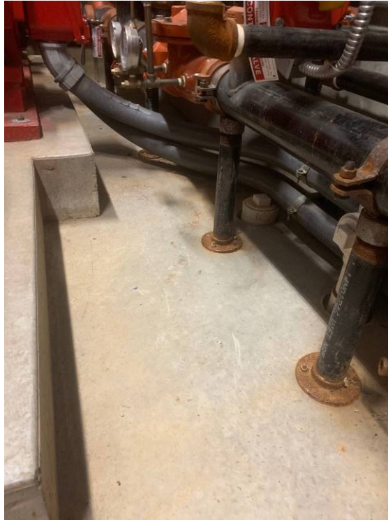
Photograph 9: Interior Pump Room B
