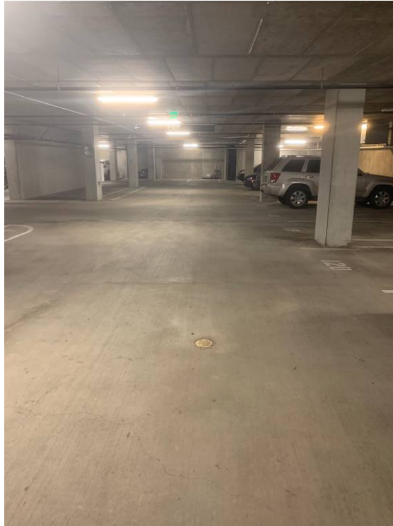
Photograph 3: Parking Garage Slab/Foundation B
