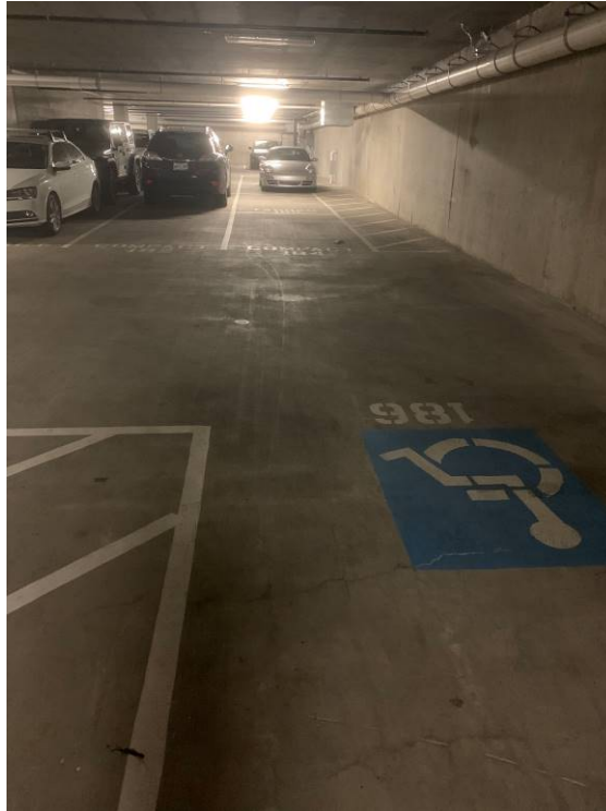
Photograph 5: Parking Garage Slab/Foundation D
