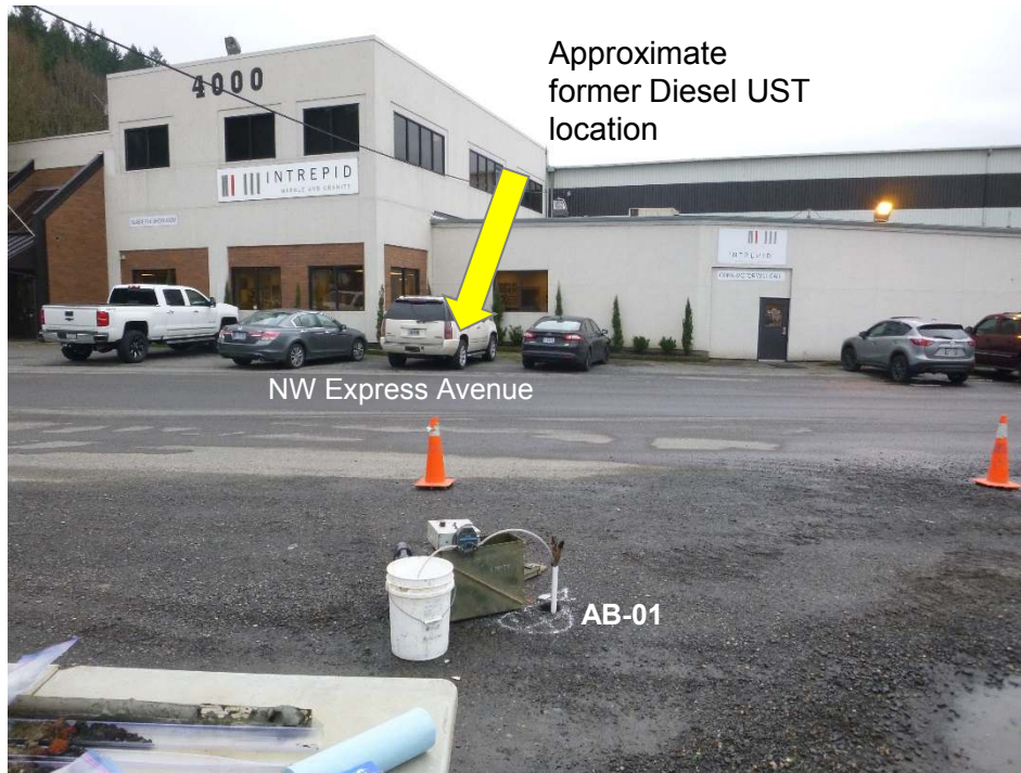
Temporary boring and groundwater monitoring point AB-01, view to the northwest. January 29, 2018
