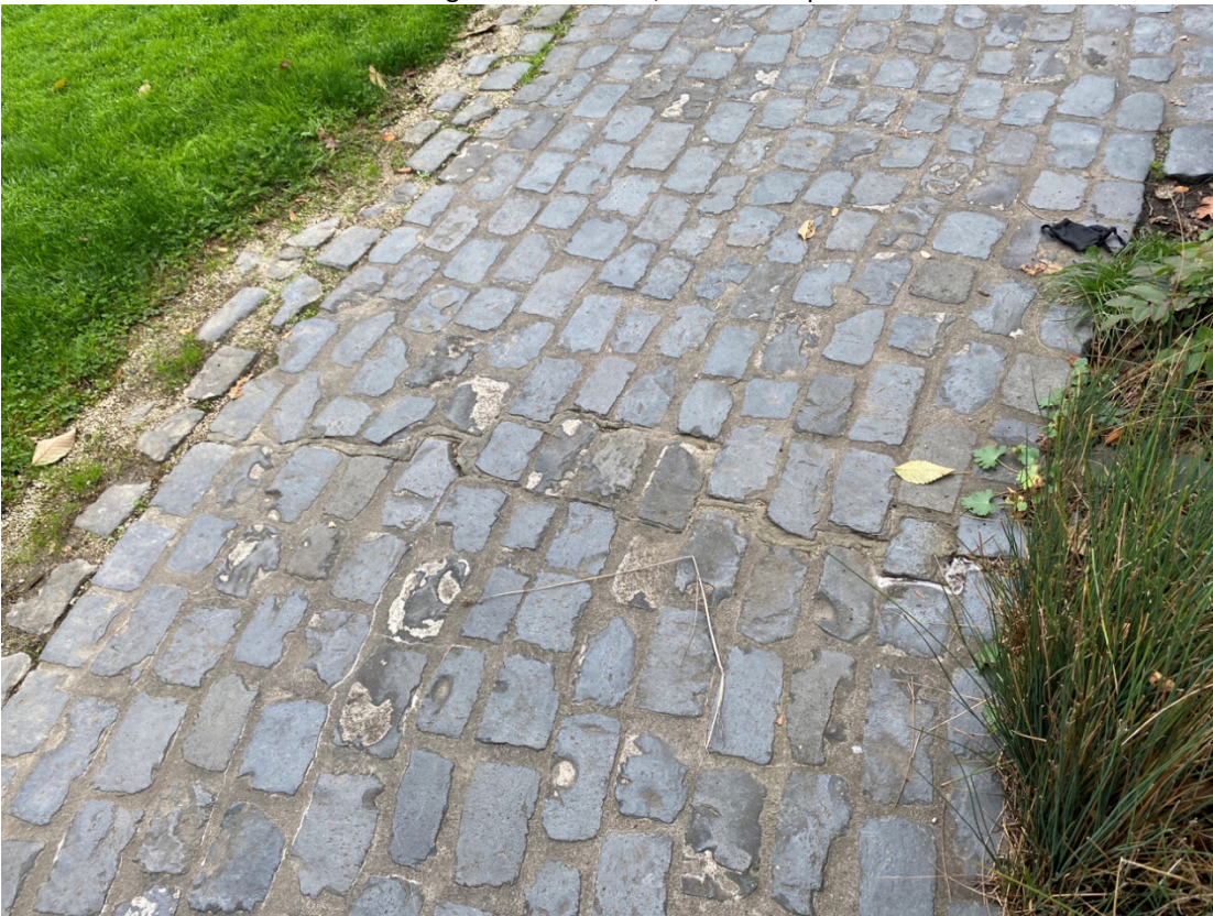
Photo Point 8 – Caulking in fair condition, does not expose subsurface soil.
