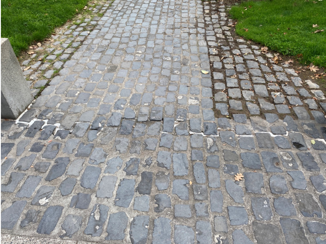
Photo Point 8 – Caulking in fair condition, does not expose subsurface soil.
