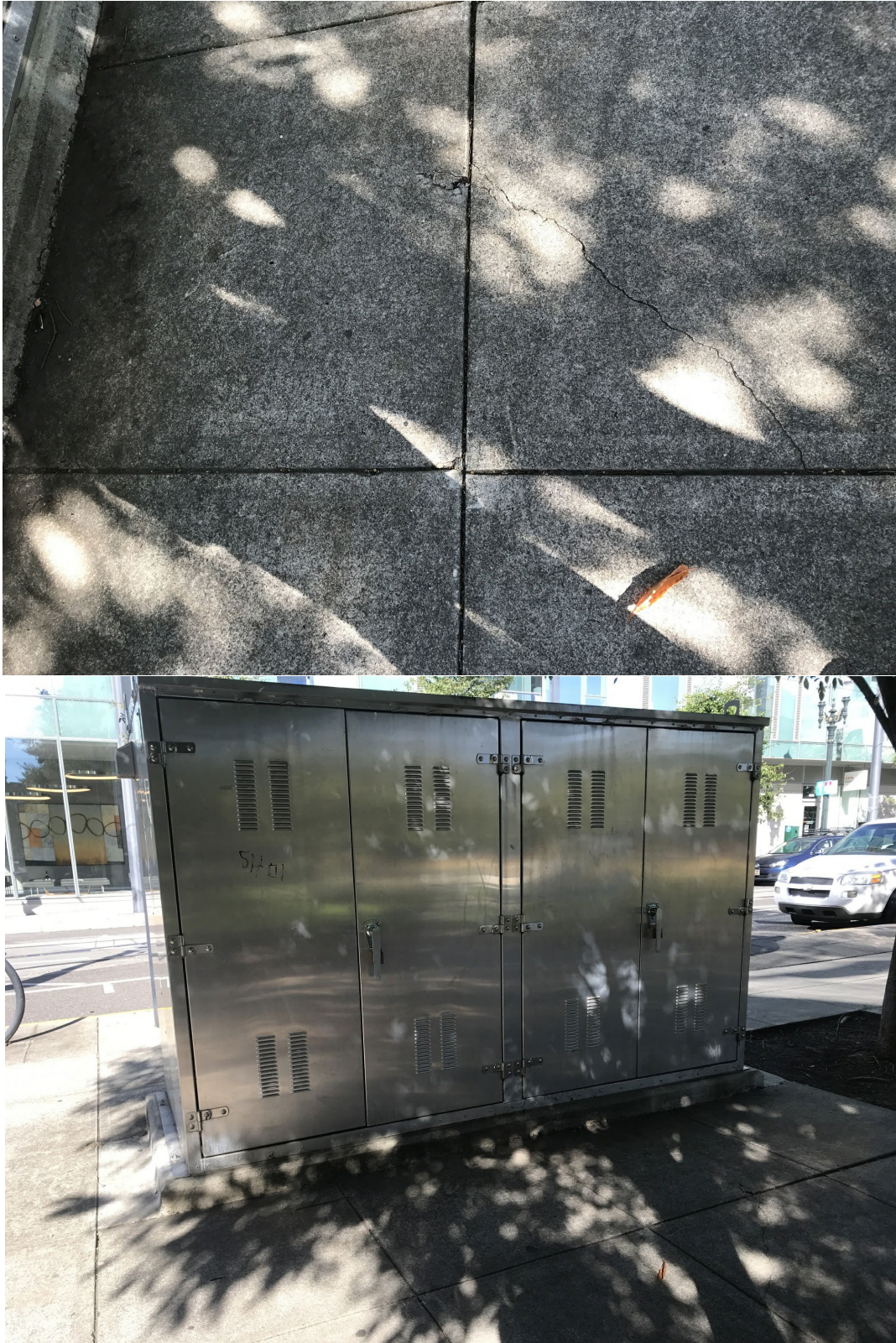
Photo Point 9 (2 photos) – (top photo) crack in panel on right has not changed since 2019 inspection. New crack has formed in the panel on the left. (bottom photo) electrical utility vault, likely for streetcar, adjacent to minor cracks in pavement shown in top photo.
