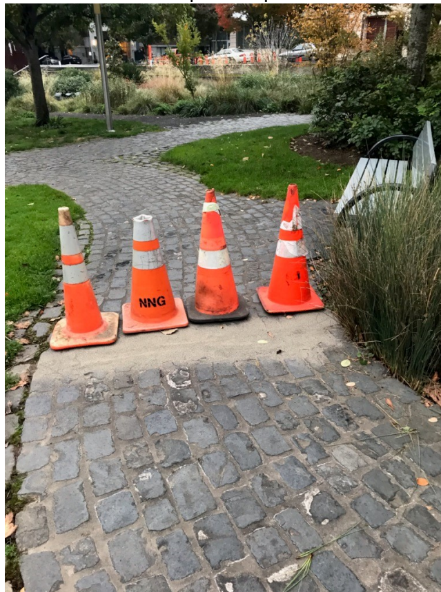
Photo Point 10 – separation of landscaping cobbles. Appeared to have previously been patched with caulking. Patch mostly gone now. No holes into subsurface observed here. Photos of the repair are provided below.
