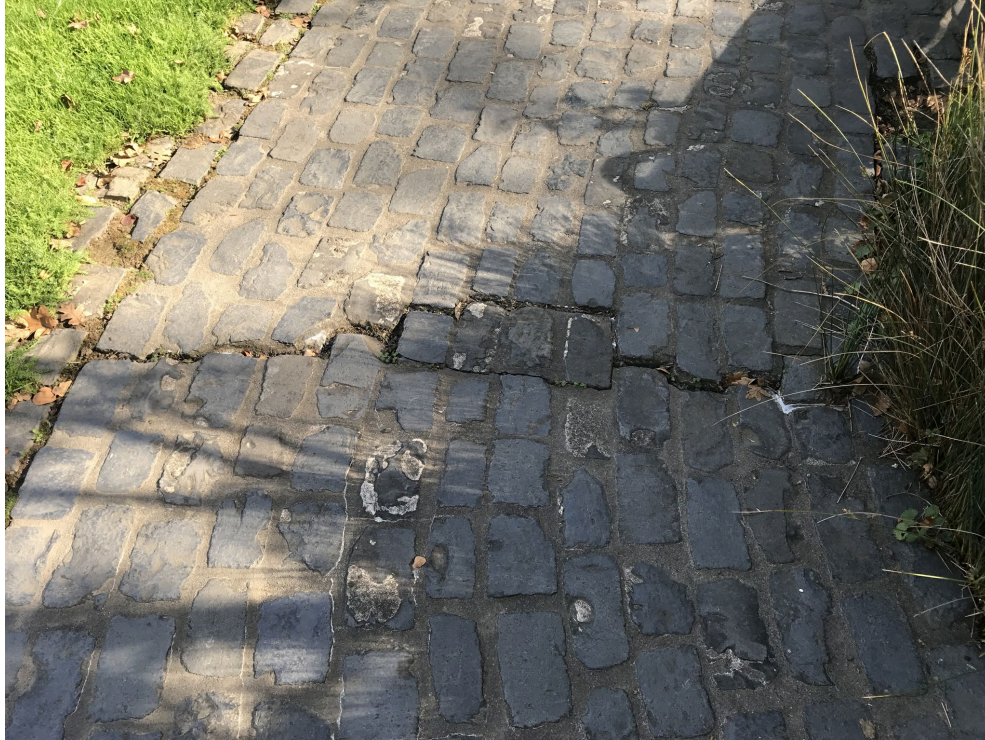
Photo Point 10 – separation of landscaping cobbles. Appeared to have previously been patched with caulking. Patch mostly gone now. No holes into subsurface observed here. Photos of the repair are provided below.
