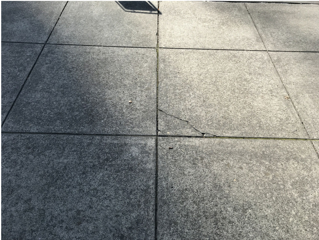
Photo Point 4 – Minor crack in pavement has not changed since last year
