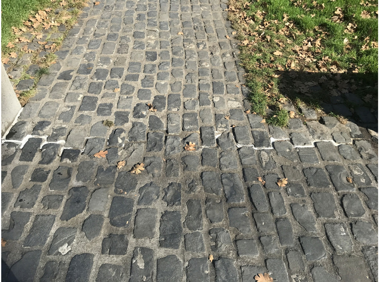
Photo Point 12 – Third location where separation of cobbles patched. This patch is in decent shape.
