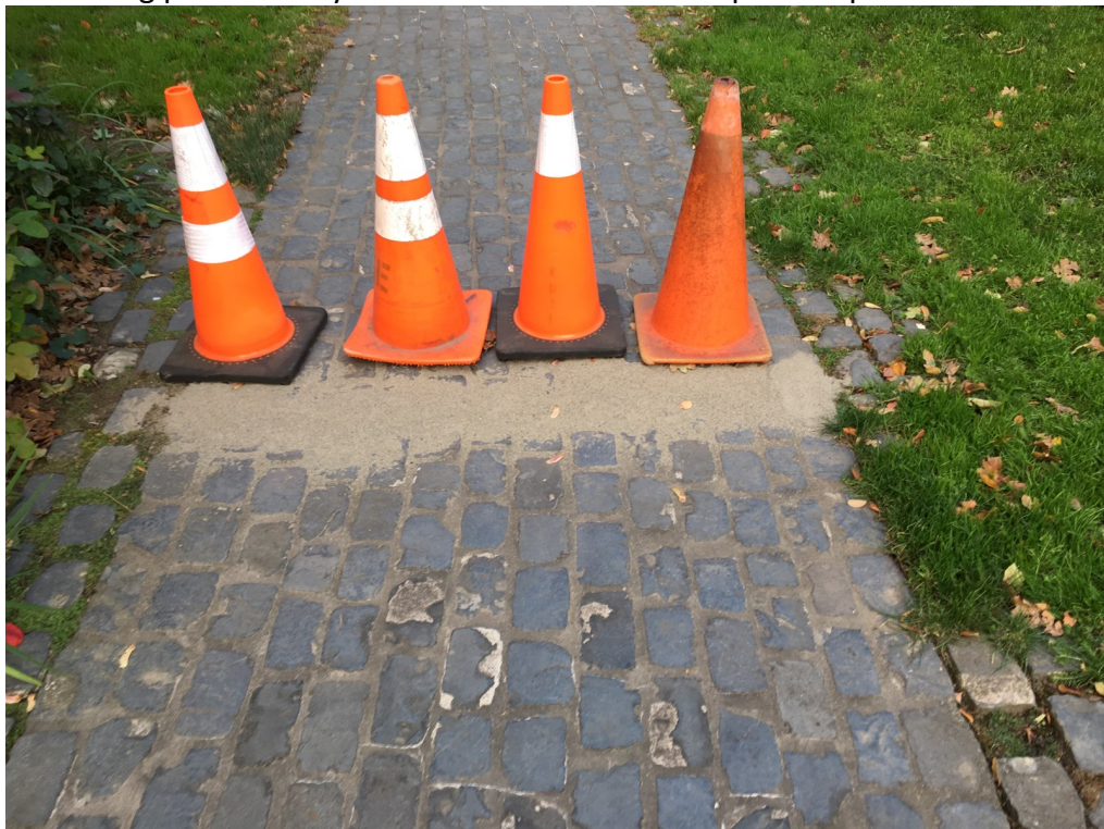
Photo Point 11 – Another location where separation of landscaping cobbles was observed. Caulking patch mostly still there. Photos of the repair are provided below.
