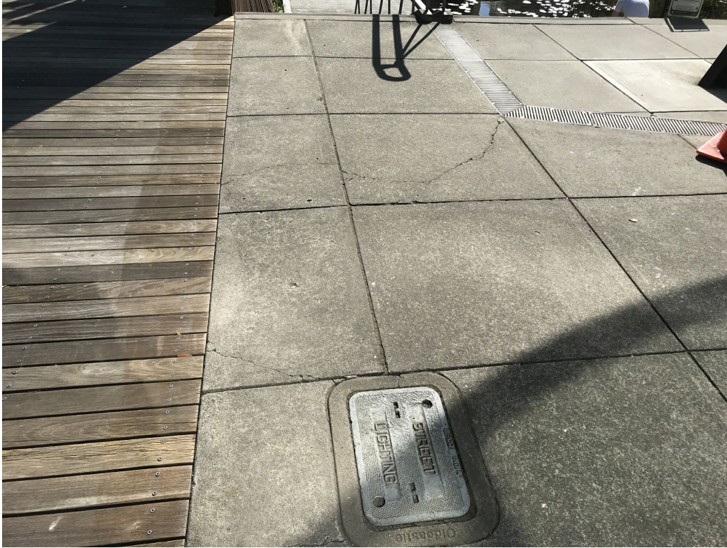
Photo Point 1 – Minor cracks in concrete pavement looks the same as it did during last year's inspection.
