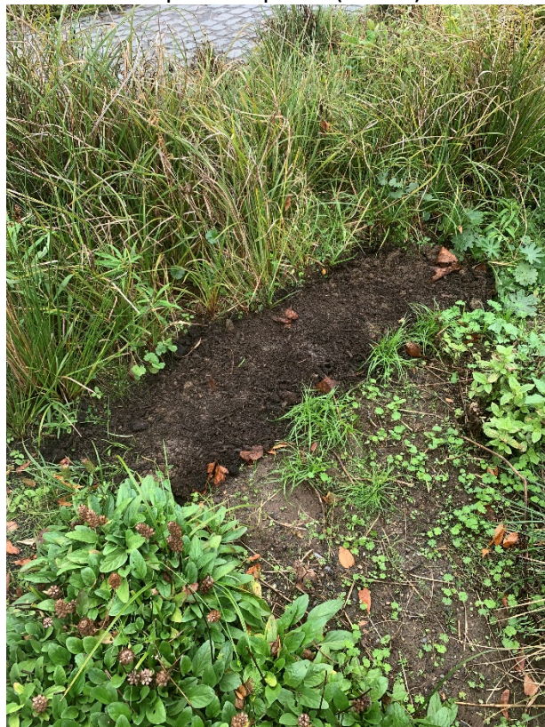
Photo Point 13 – Area of surface erosion. Thick black material observed at the surface (above) Repair soil patch (below)
