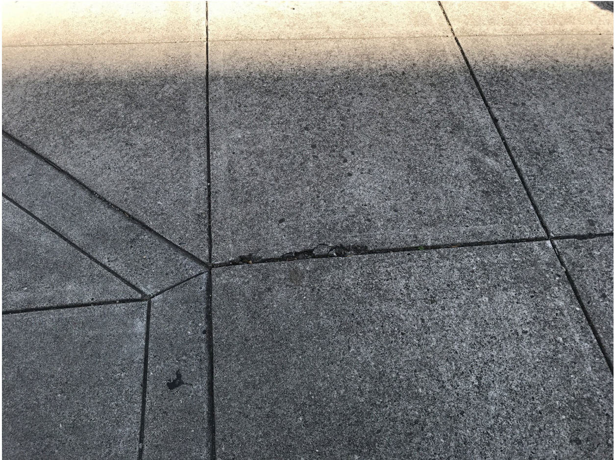
Photo Point 8 – Minor wear at panel edge.
