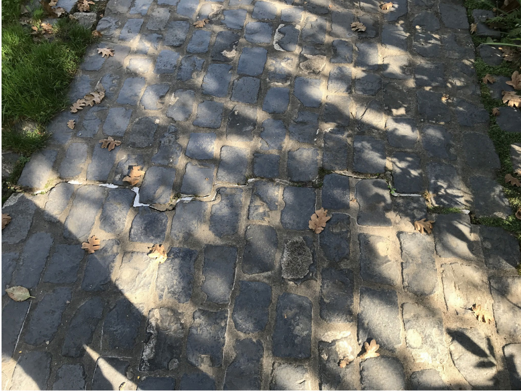
Photo Point 11 – Another location where separation of landscaping cobbles was observed. Caulking patch mostly still there. Photos of the repair are provided below.
