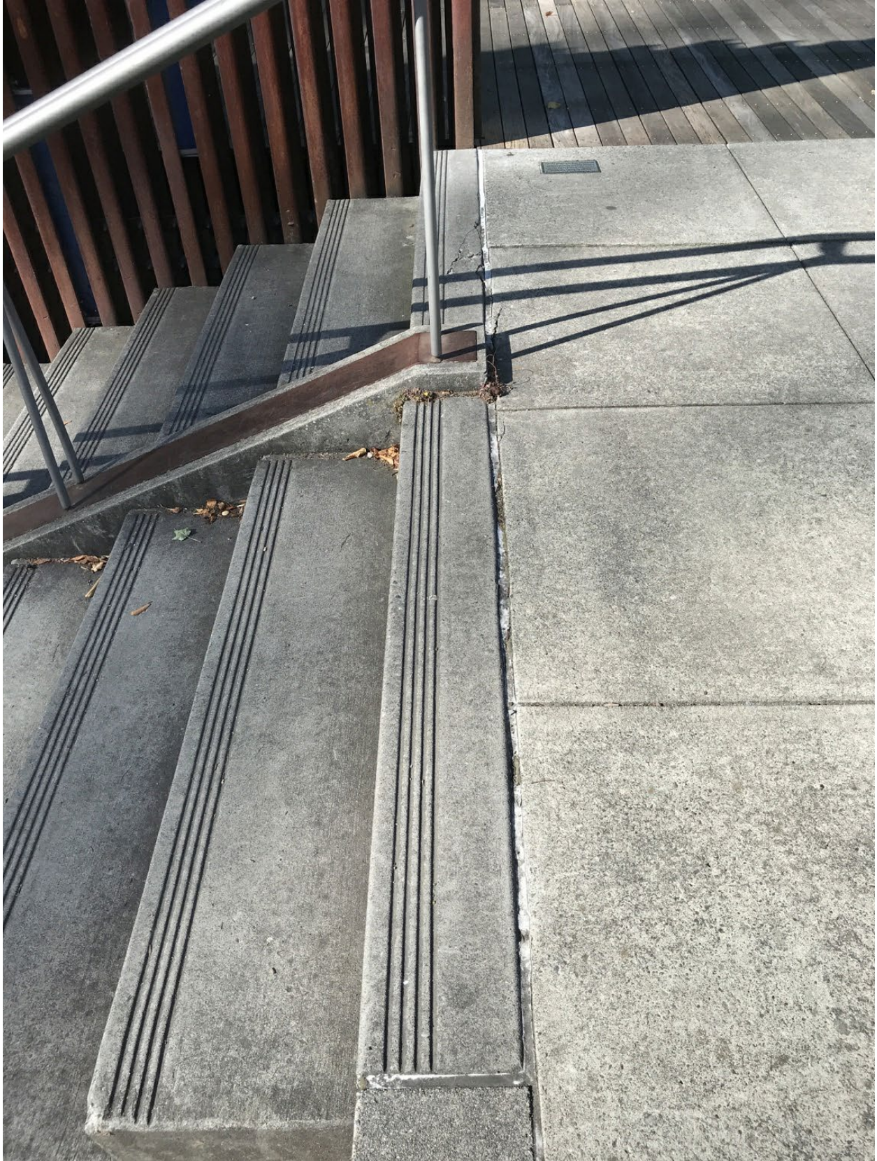
Photo Point 5 – Minor cracks in pavement at top of staircase
