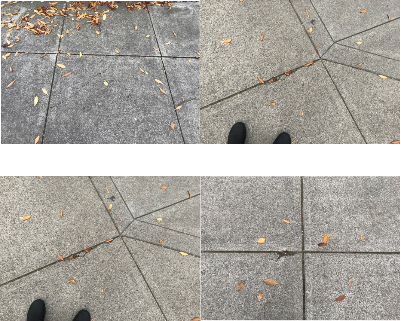
Photos 1-4 : Minor cracking in concrete panels
