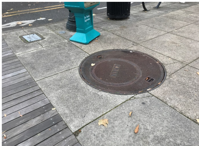
Photos 5-8 : Minor cracking in concrete panels
