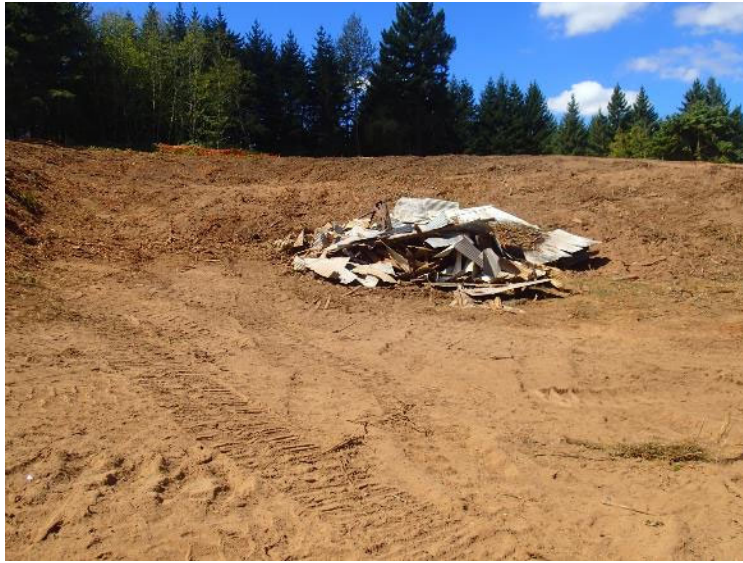
Demolition debris was gathered and disposed of or recycled (August 31, 2017).
