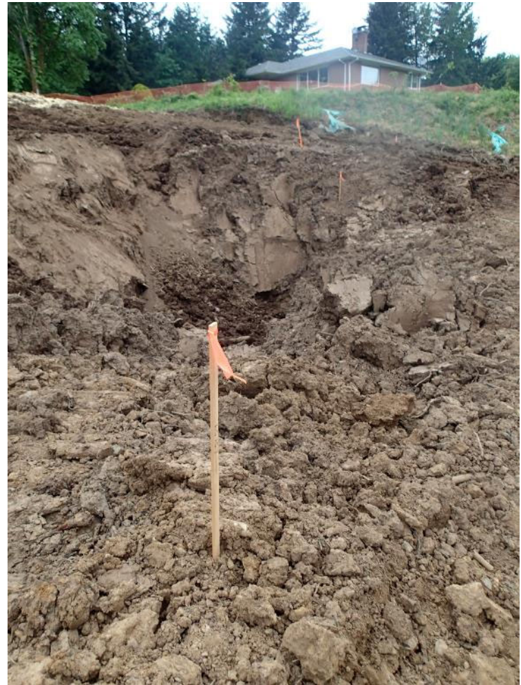
Close-up showing 3-foot-minum soil cap along western landfill boundary (May 17, 2018).
