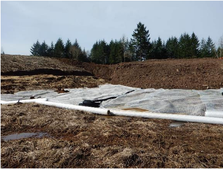
View west showing the buttress fill (left) and demarcation grid and cap (right). Note cap is substantially > 3 feet thick (March 29, 2018).
