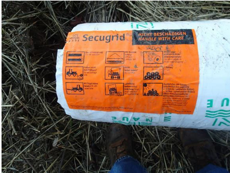
A roll of demarcation grid (geotextile) to be placed over the landfill footprint prior to installing cap (February 12, 2013).
