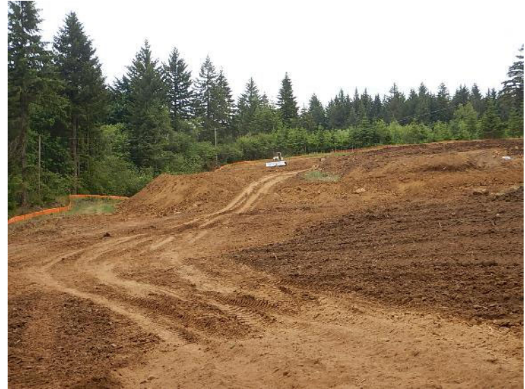
South buttress fill (June 7, 2018).
