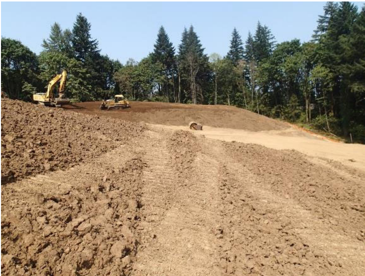
North buttress fill on August 22, 2018.
