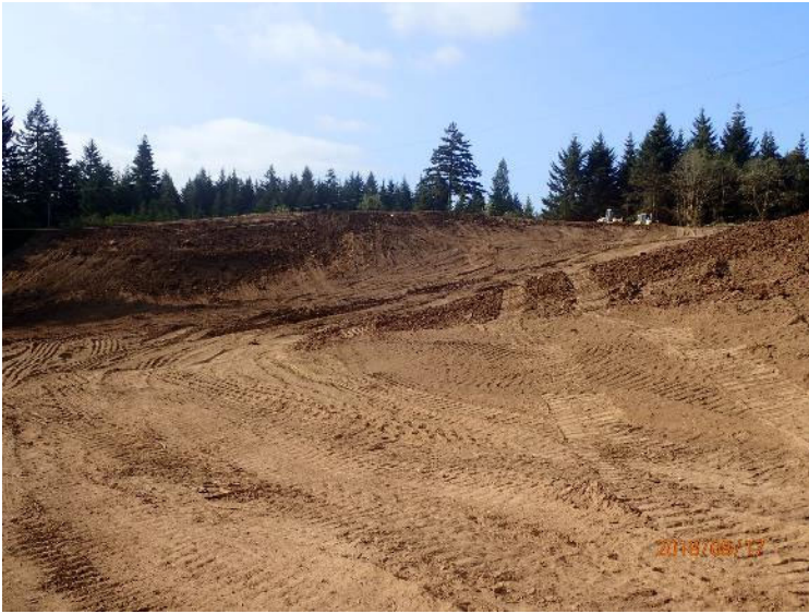
South buttress fill on August 17, 2018.
