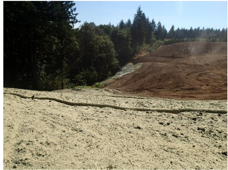
North buttress fill was hydroseeded and straw wattles placed according to erosion and sediment control plan (August 29, 2018).
