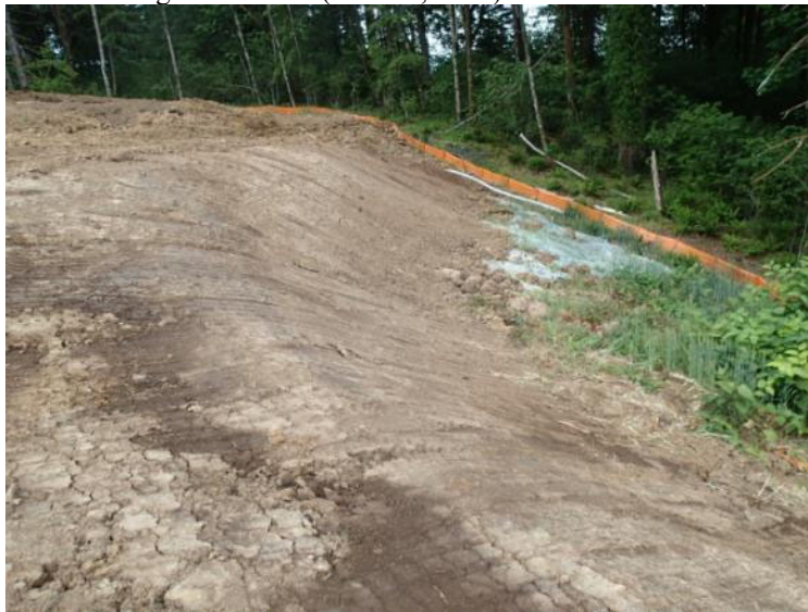
Cap over the eastern landfill boundary – view north (June 14, 2018).
