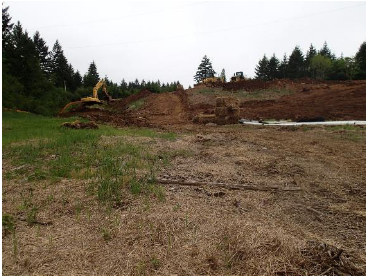
Keyway excavation of south buttress (May 17, 2018).
