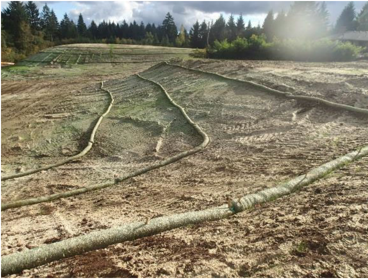
Straw wattles were placed on the remaining portions of the landfill, after which the ground surface was hydroseeded— view south (October 9, 2018).
