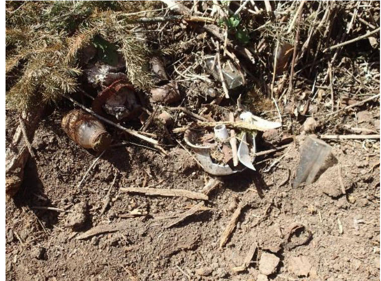
De minimis quantities of solid waste exposed at the ground surface were not removed since the entire landfill would be capped with 3 feet of soil.
