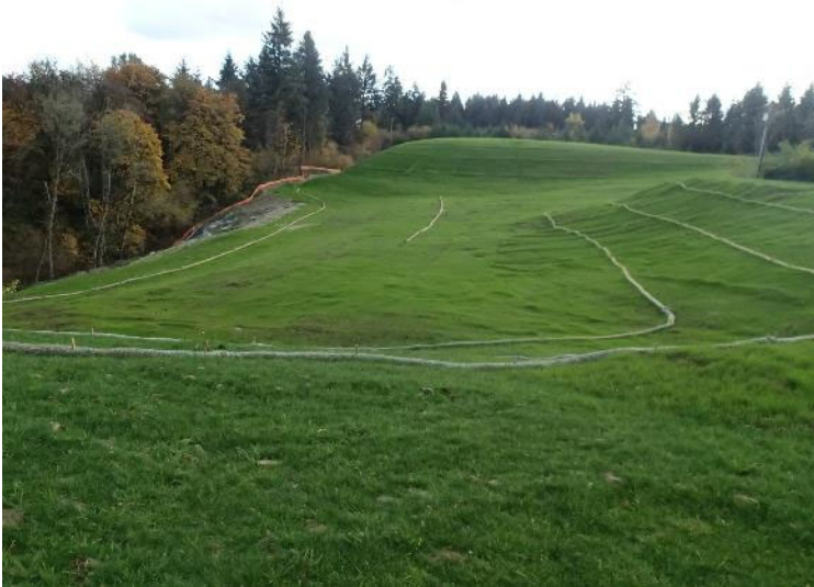
Grass has taken root over the capped landfill and buttress fills – view south (November 6, 2018).
