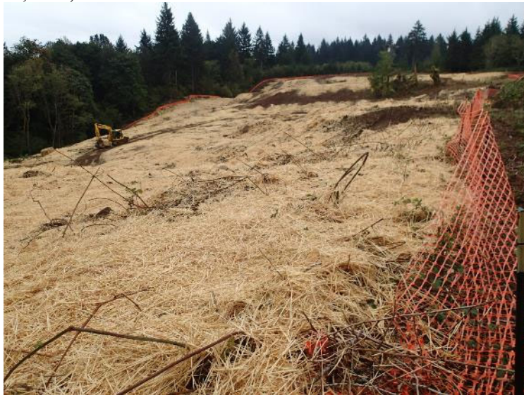
Straw was placed over the soil surface for erosion control purposes – view south (September 29, 2017).
