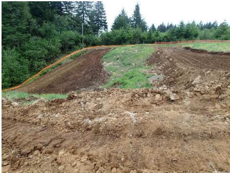
South buttress keyway (left) and bench (right) as seen on May 17, 2018).
