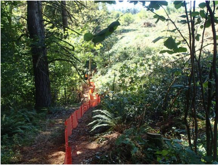
A silt fence was installed around the perimeter of the disturbed area – view of east boundary looking south (August 16, 2017).
