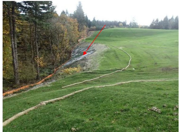
Rip-rap is being considered to cap the steep, eastern margin of the landfill where the demarcation grid is still visible.
