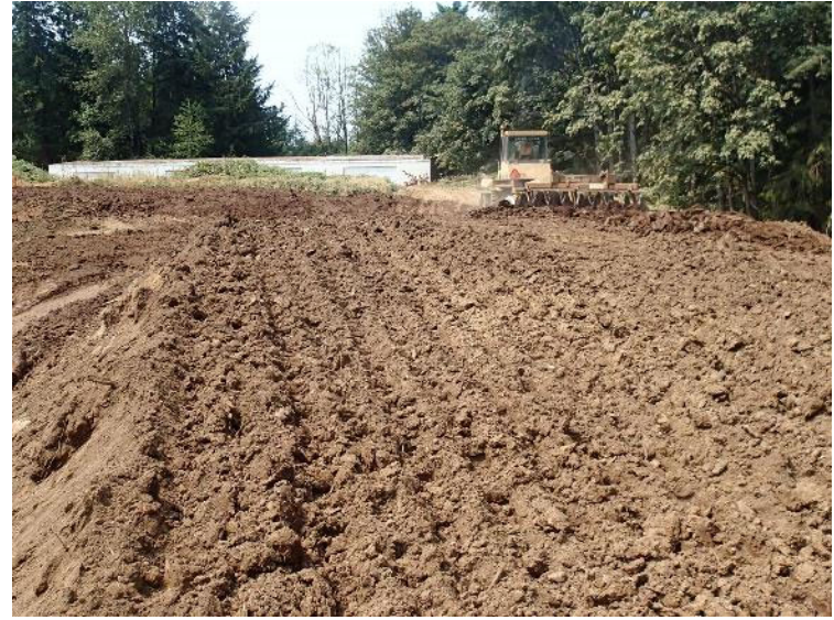
North end of landfill cap being prepared for seeding.
