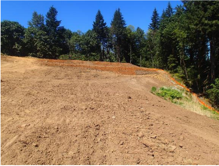
North buttress fill (July 24, 2018).
