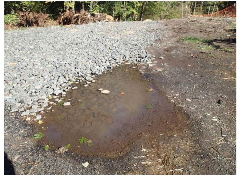
Rock was placed over the haul routes on the upslope west side of the landfill (October 13, 2017).
