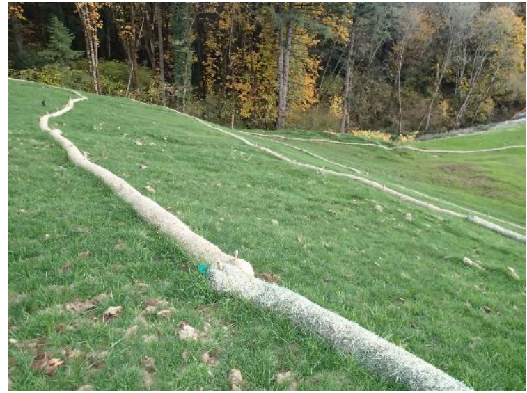
North buttress fill – view east (November 6, 2018).
