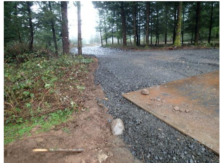
Gravelled haul road west of the landfill (January 18, 2018).
