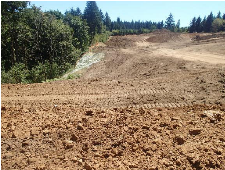
South buttress fill (under construction) from the perspective of the north buttress (July 24, 2018).
