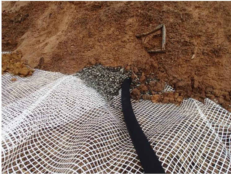
Drain pipe were bedded and covered with gravel prior to placing the soil cap (March 2, 2018).
