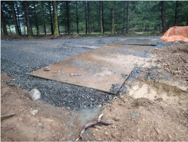
Steel plates positioned at unloading platform at the west margin of the landfill (January 18, 2018).
