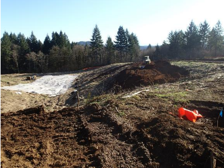
Construction of the buttress fill south of the landfill (right side of the demarcation represents the southernmost extent of the landfill) – view southeast (February 12, 2018).
