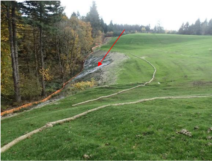
Area where rip-rap was proposed to cap the steep, eastern margin of the landfill where the demarcation grid is still visible.
