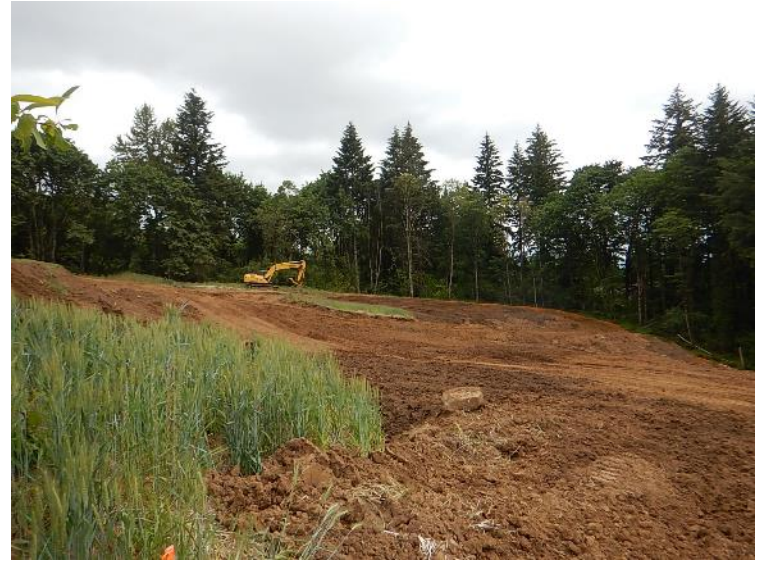
View north of cap at the north end of the landfill (June 7, 2018).
