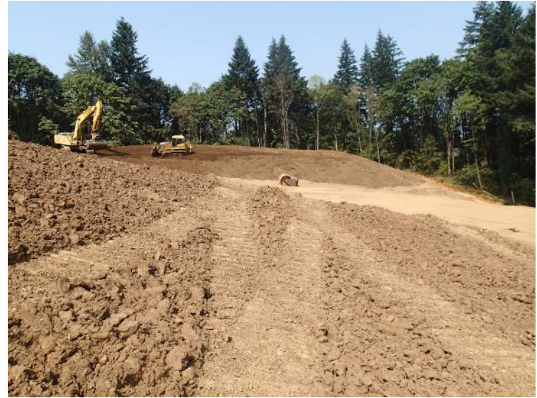
North buttress fill on August 22, 2018.
