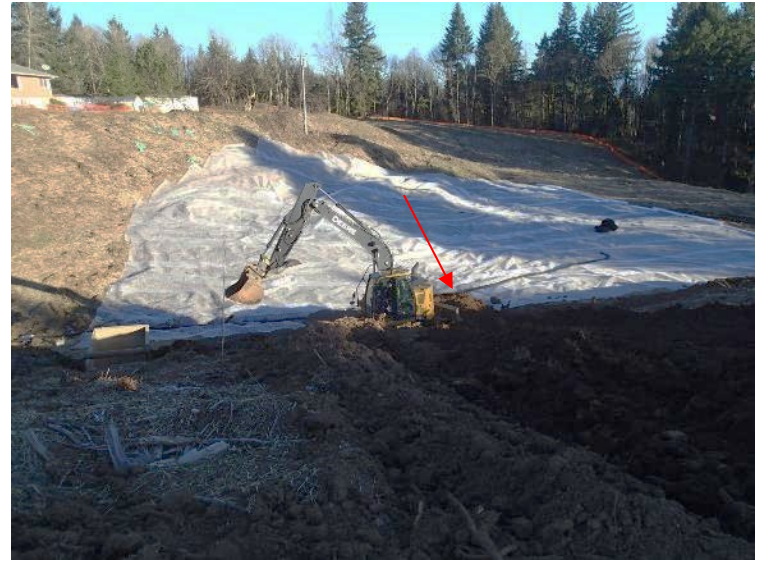
Demarcation placed over southwest corner of landfill. Note drain pipe placed along centerline of ravine – view north (February 13, 2018).
