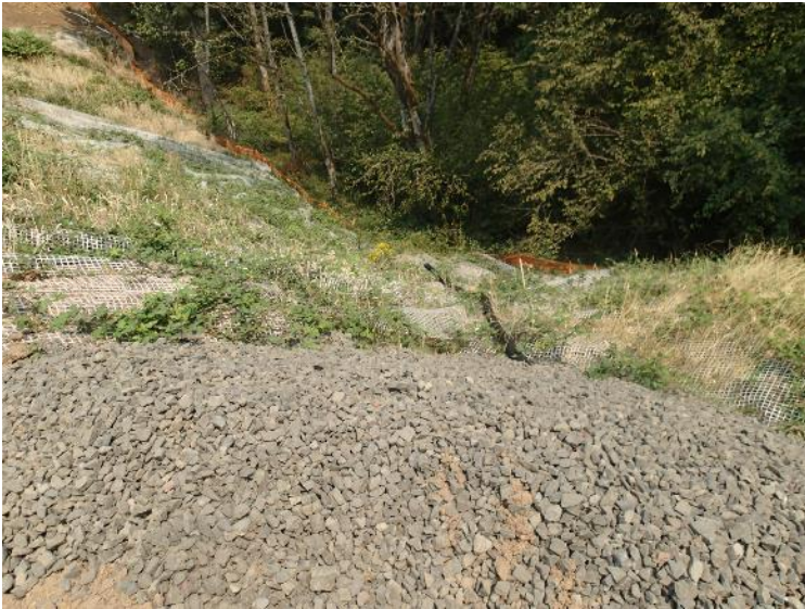
Drain rock was placed over the ravine drain line. Drain pipe exits at the eastern landfill boundary, which has not yet been capped as of this date (August 8, 2018).
