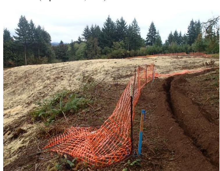
Water line to an east-adjacent residence was diverted around the landfill (October 13, 2017).
