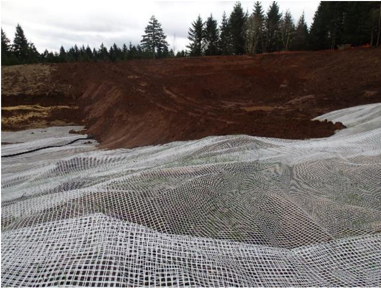
View south of buttress fill and soil cap beginning to be installed above the demarcation grid (March 2, 2018).
