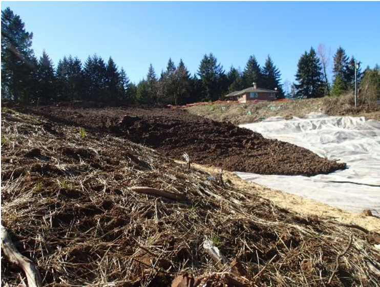
Continued cap installation over the demarcation grid on the southwest part of the landfill – view northwest (March 3, 2018).
