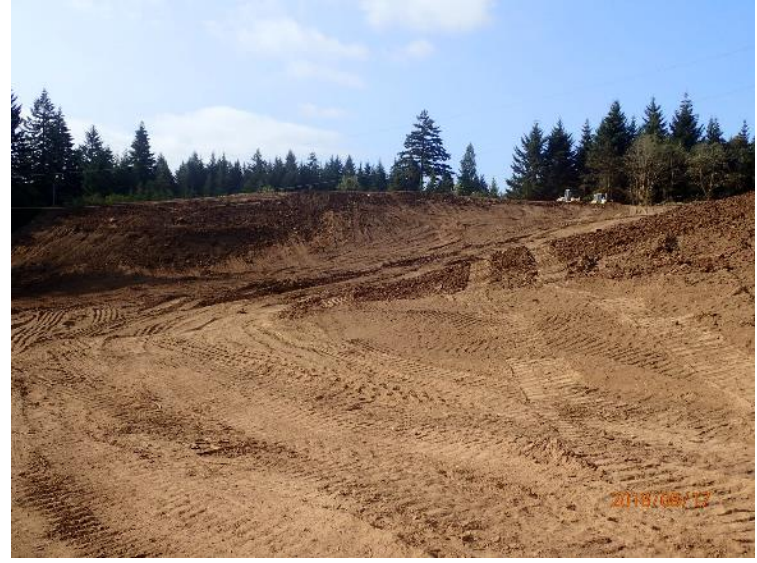
South buttress fill on August 17, 2018.
