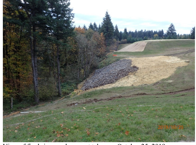
View of final rip-rap placement taken on October 25, 2019.
