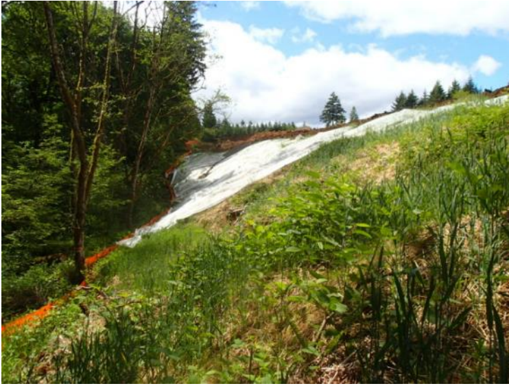
Demarcation grid installation along the east-central edge of the landfill - view south (June 1, 2018).
