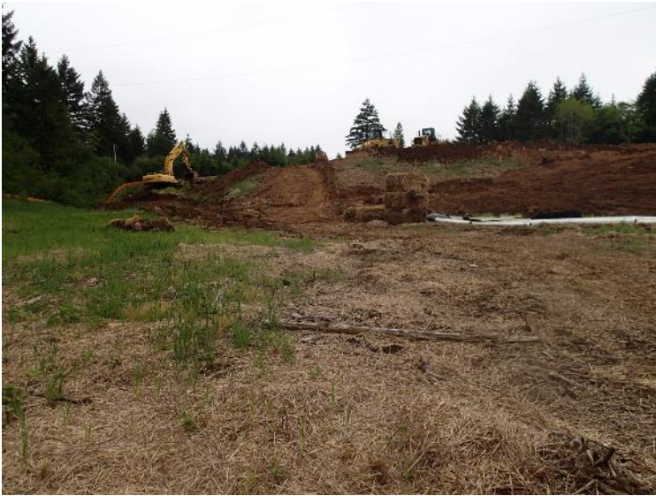
Keyway excavation of south buttress (May 17, 2018).
