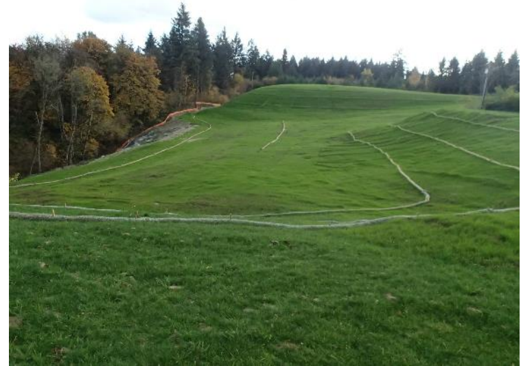
Grass has taken root over the capped landfill and buttress fills – view south (November 6, 2018).
