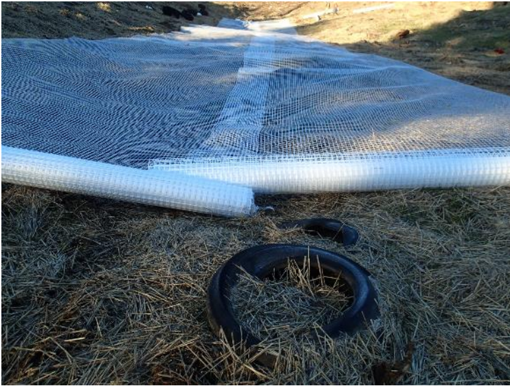
Close-up photo showing the overlapped demarcation grid – view west (February 12, 2018).
