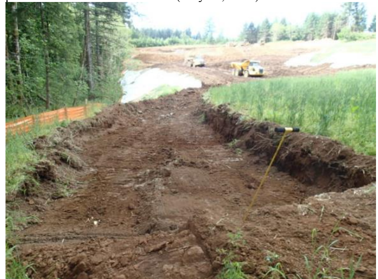
Keyway excavation along the east side of the north buttress fill - view south (June 1, 2018).
