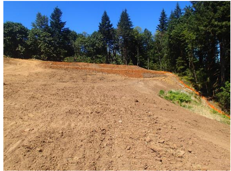
North buttress fill (July 24, 2018).
