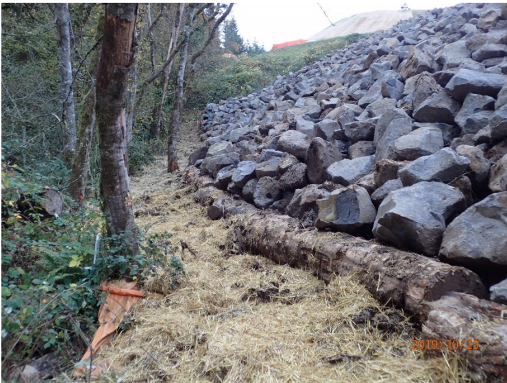
Logs secure and stabilize the downslope margin of rip-rap.
