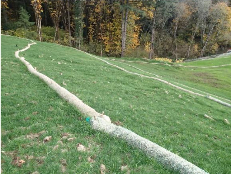
North buttress fill – view east (November 6, 2018).
