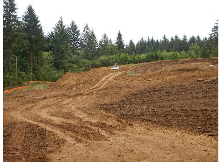
South buttress fill (June 7, 2018).
