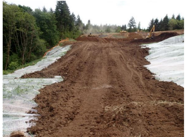
Soil cap being installed over the demarcation grid at the east-central part of the landfill – view south (May 30, 2018).
