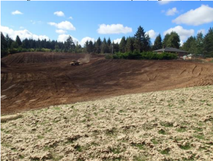
Grass has taken root on the north buttress fill, and the remainder of the landfill is being prepared for hydroseeding (September 14, 2018).
