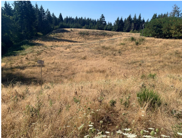
View south across landfill cap showing summer season grass cover stabilizing slope conditions.
