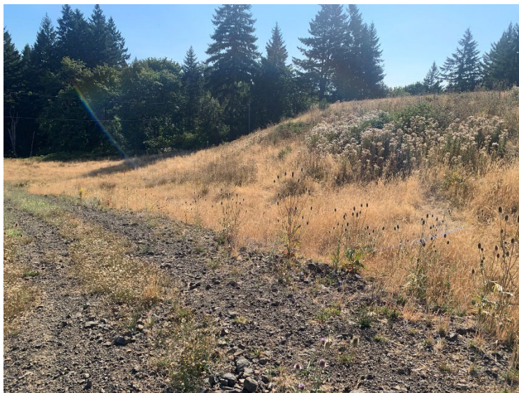
View east showing access road from the former south truck entrance and south buttress slope.
