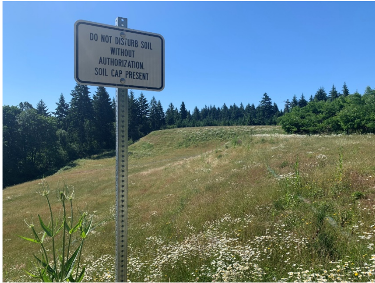
View south across landfill cap showing summer season grass cover to provide stability of slope conditions.
