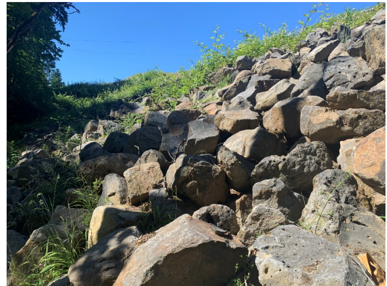
Closer view of landfill toe cap showing riprap with large logs at the toe.
