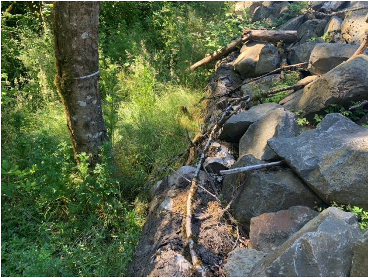
Toe of rip rap slope, looking south.
