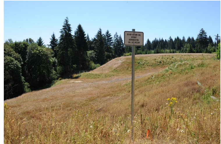
Signs have been posted at the perimeter of landfill cap to warn against unauthorized digging.
