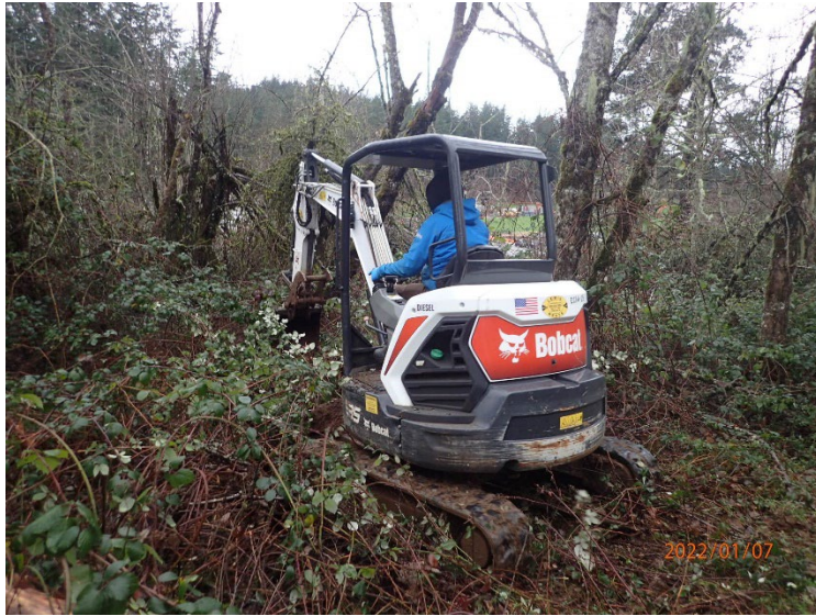
A mini excavator assisted with the collection of ISM subsamples by clearing a pathway into heavily vegetated areas of DU01.
