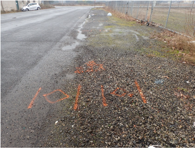
View of utilities identified along SE Powell Valley Road.
