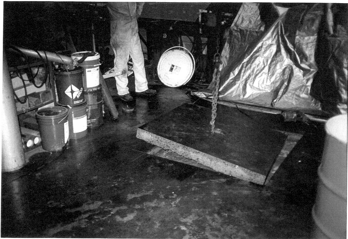
Beginning 1999 w/o UST Decommissioning
