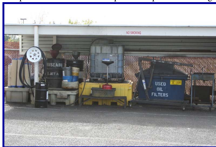
Used oil and sump fuel ASTs with secondary containment pallet adjacent waste fuel drums.
