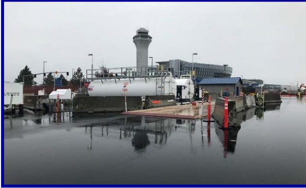
North Fueling Station
