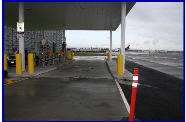
South Reload Rack.
