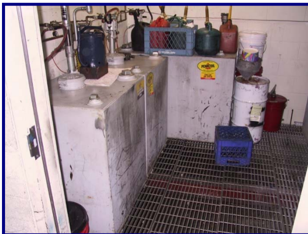
POL storage building with secondary containment.
