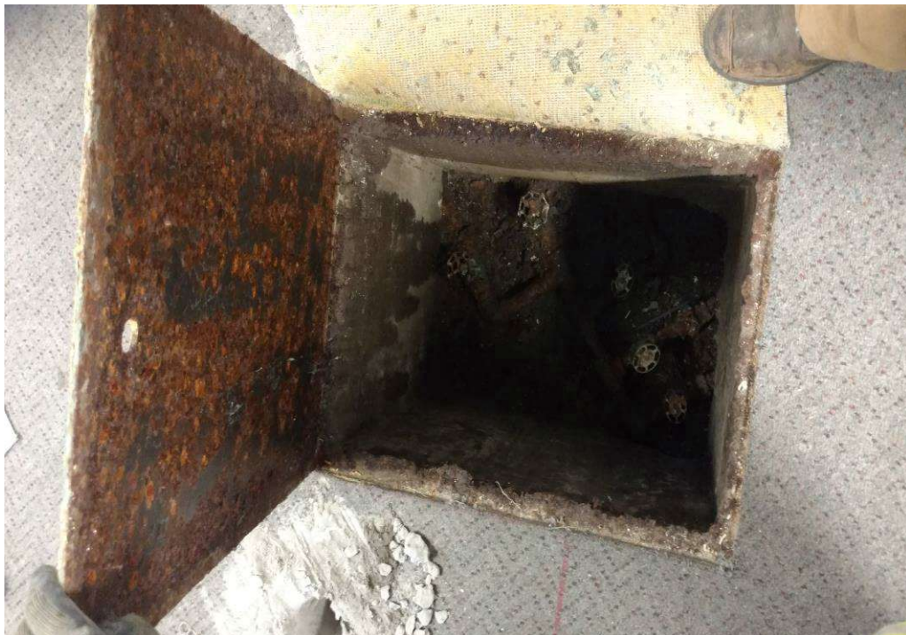
Photo 2 View of the suspect former waste pit / valve box located inside the Goodwill building.
