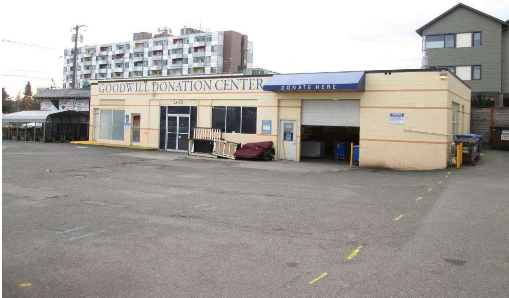
Photo 1 General view of the existing Goodwill building and former auto service facility at the site.
