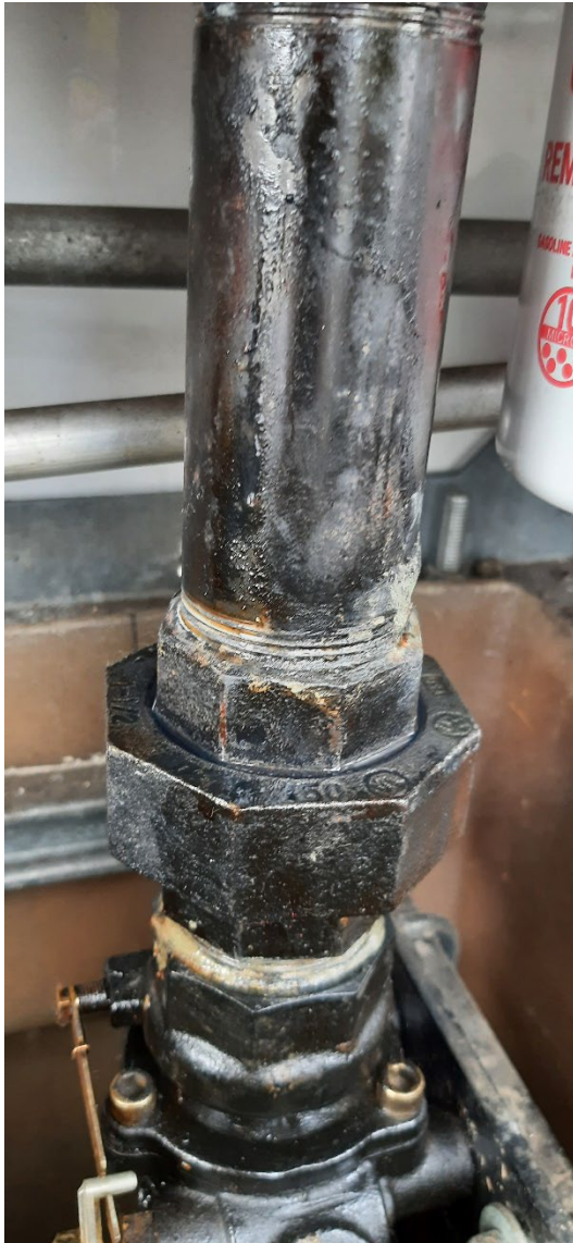
9: Weeping unlead/regular pipe in UDC #6
