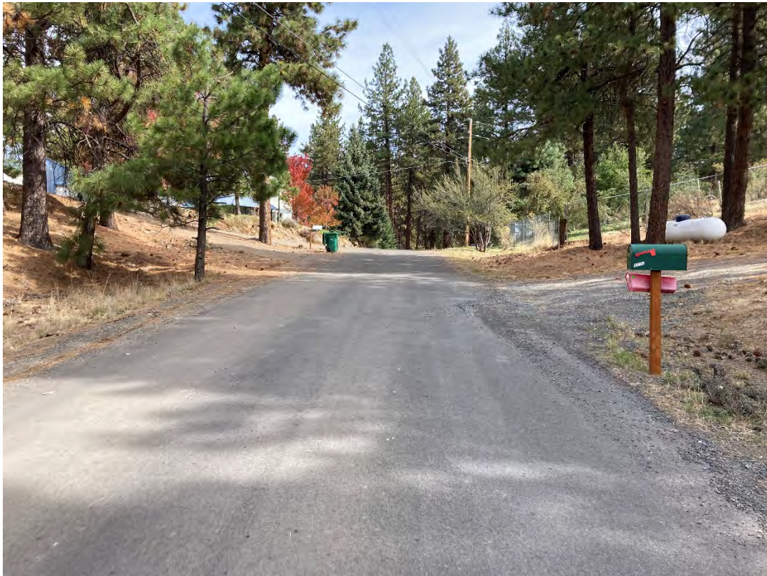
The southern end of the Thicket Court is still in better condition than the northern portion.
