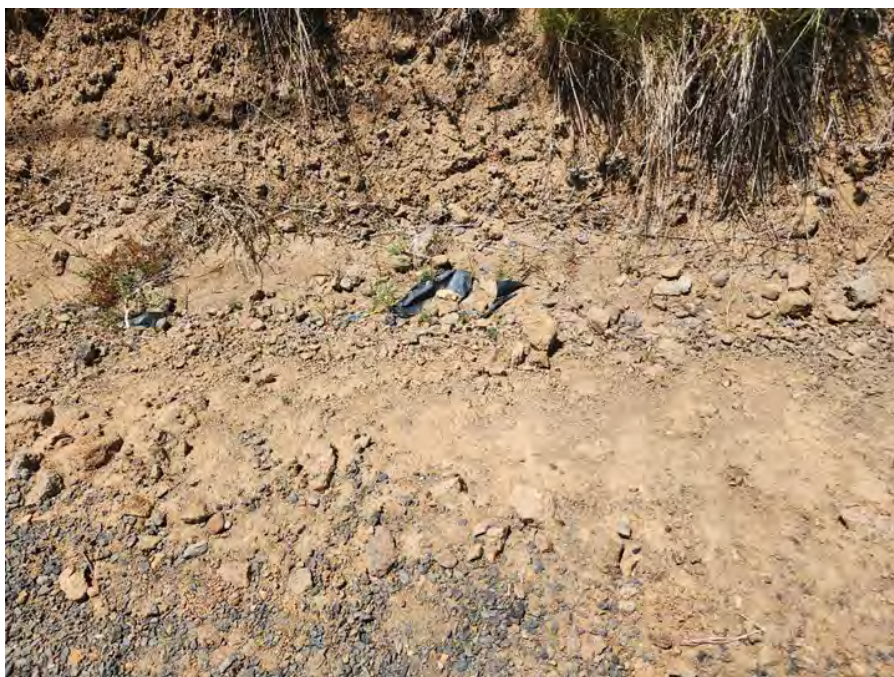
North Ridge Drive – Black Geomembrane exposed along shoulder near Parcel D.
