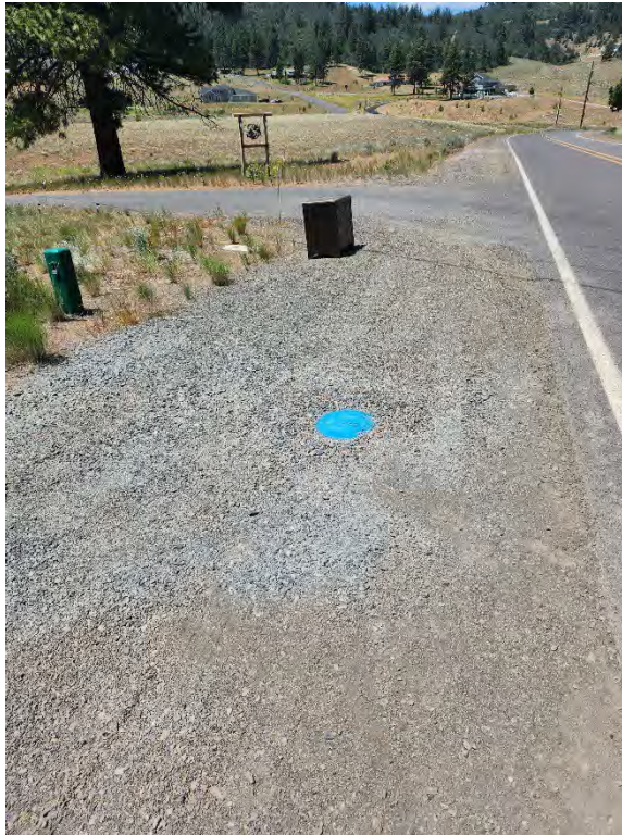
Old Fort Road – View of recently repaired area of gravel shoulder.
