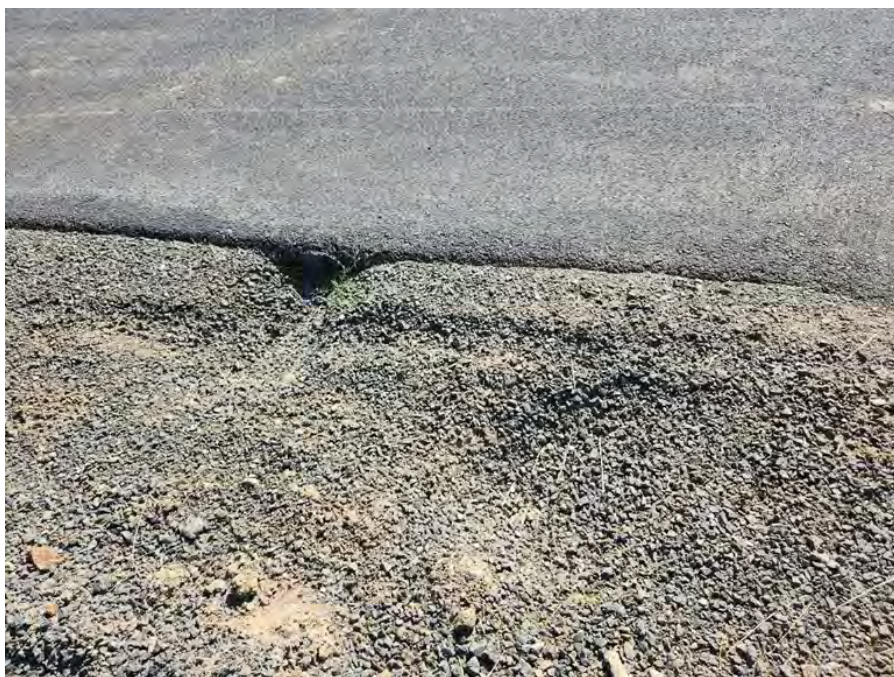
North Ridge Drive – View of depressions in gravel shoulder.
