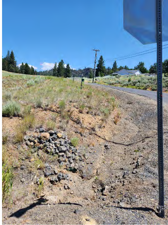
Scott Valley Drive – View from Southwest corner of road where erosion in ditch is present (same as 2022).
