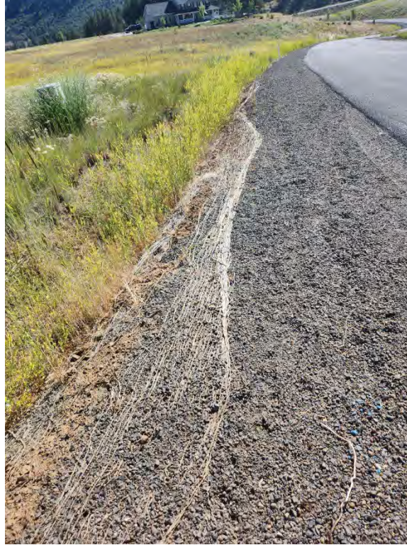
Hunter's Ridge Road – View of exposed Coconut Fiber Mat on North shoulder of road.
