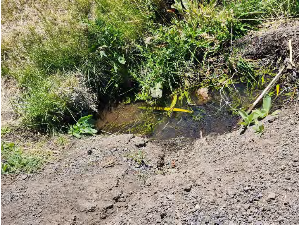
Scott Valley Drive – Standing Water located on the Southern side of the road, result of blocked culvert.
