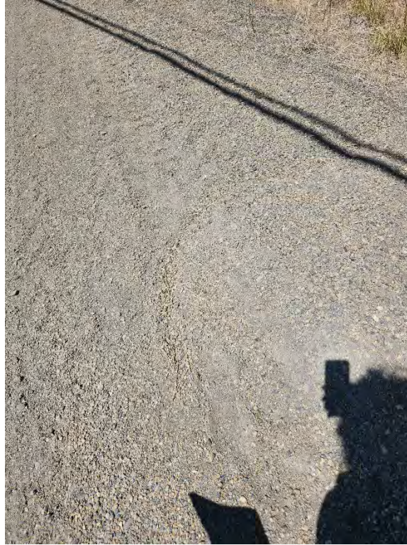
Old Fort Road – View of Rills observed on gravel shoulder.
