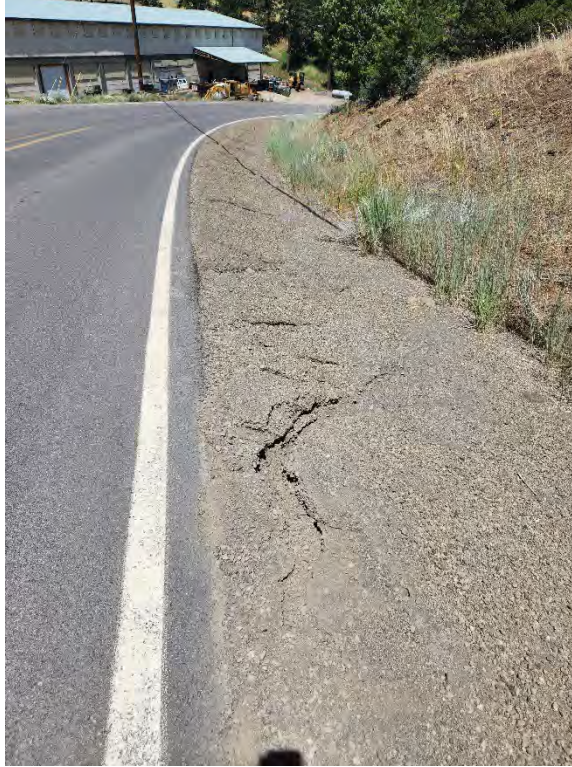
Old Fort Road – View of Gully along gravel shoulder of road.
