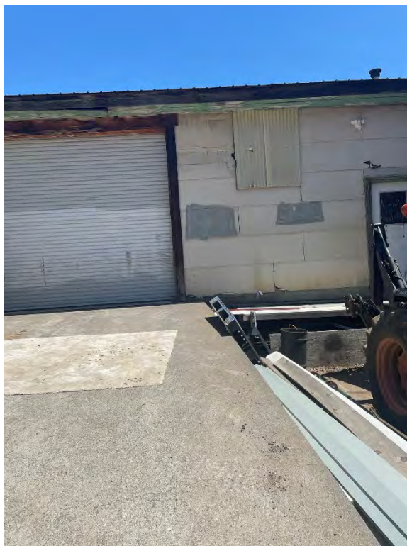
Parcel MBK-G – Suspect cement asbestos board (CAB) siding on West exterior of Warehouse.
