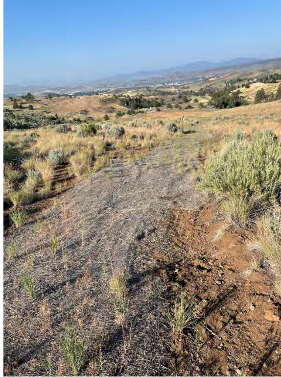
Parcel BP – Repaired gully system through parcel on the East side.
