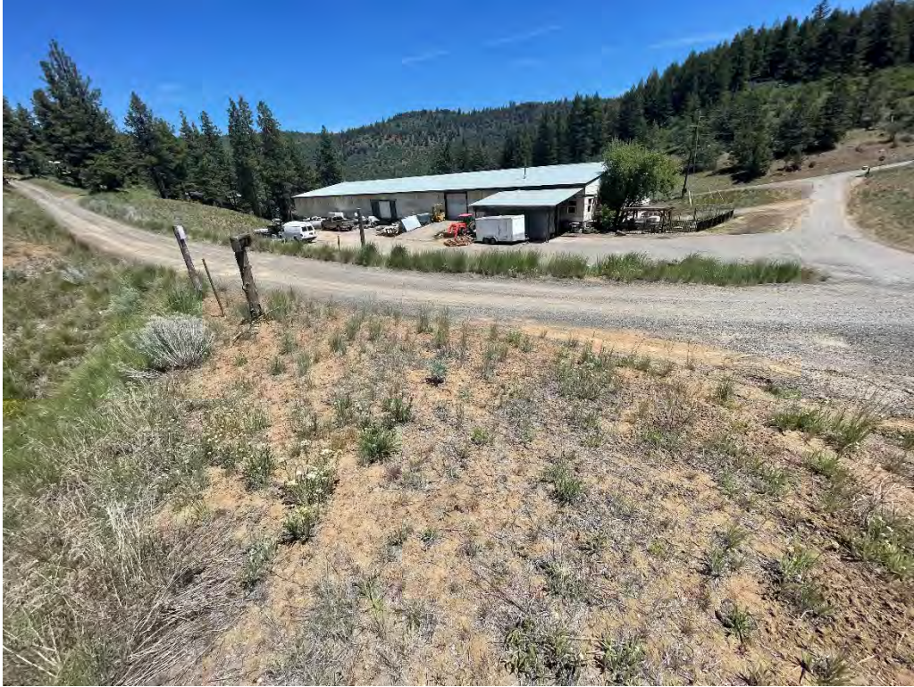
Parcel BR3 – Southwest corner of the Parcel, facing Northeast.
