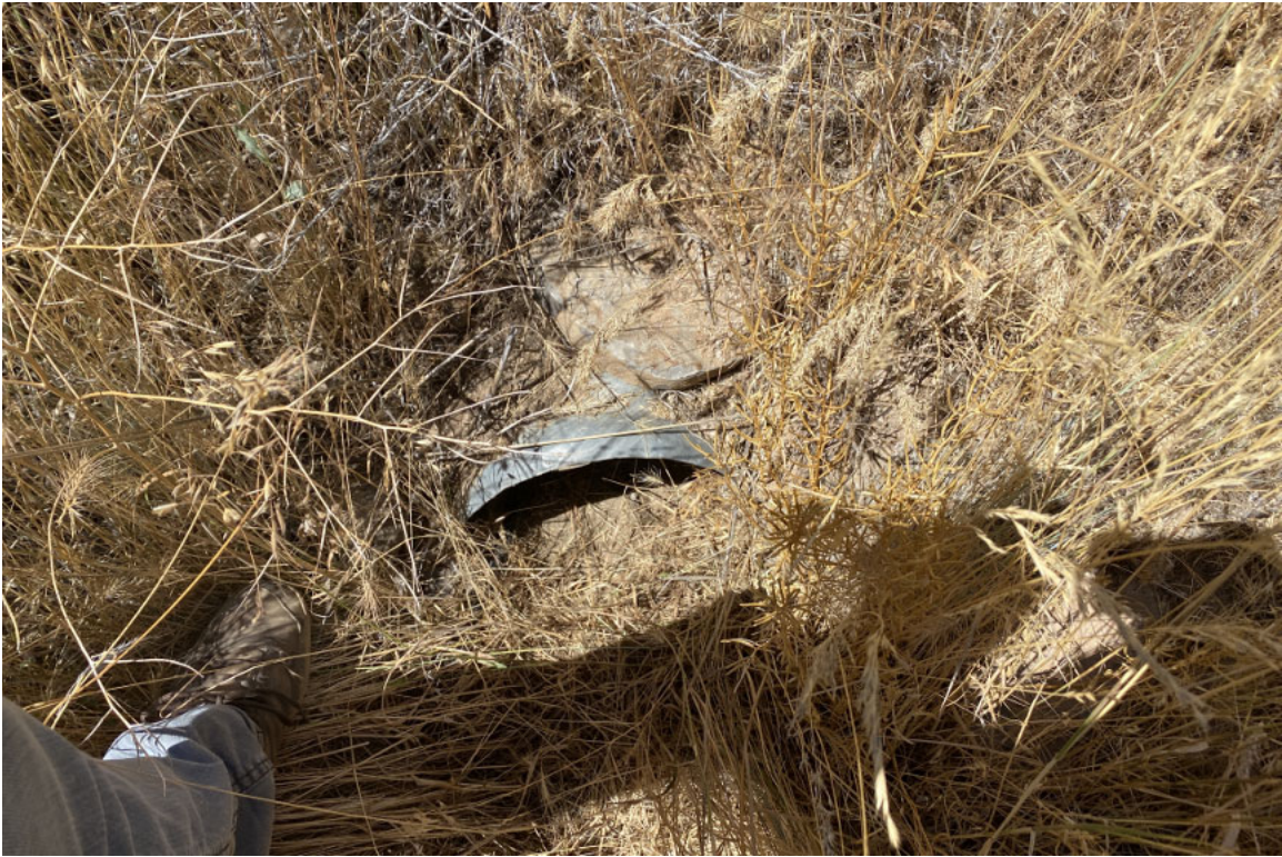
At least one of the culverts at the BR removal area was substantially blocked by sediment.
