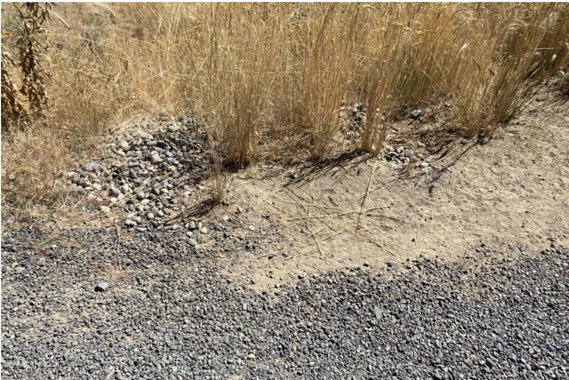
Round rock has been added in places to prevent/repair erosion locations.
