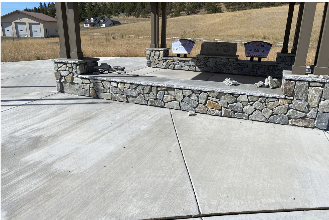
Some of the rock-work placed on the gazebo is failing and coming off the structure.
