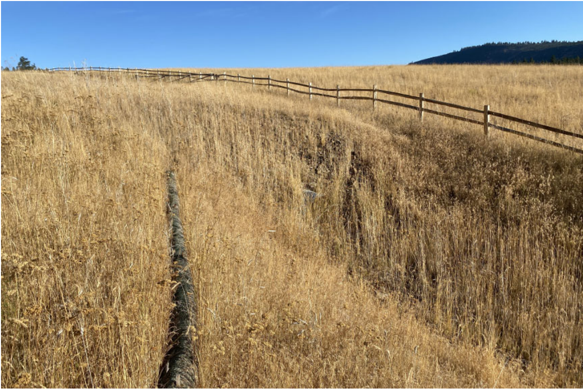
A straw wattle was located adjacent to the crest of the slope next to the southern culvert.
