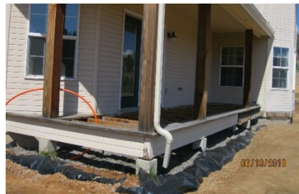
Example of Black Liner. 2018. Black liner with rock to hold in place on Parcel A.
