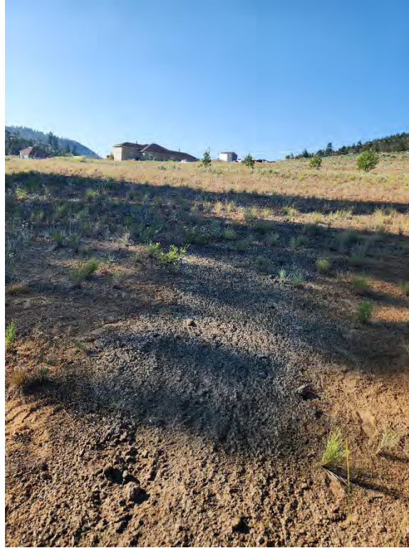
Parcel MBK-C – View of North Central portion of Parcel; repairs made in response to washout caused by frozen air valve.
