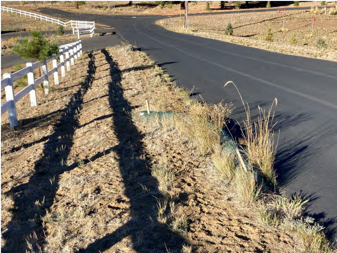
Straw wattles were present along the driveway to try and prevent erosion. Some cracking of the driveway was noted adjacent to these areas.
