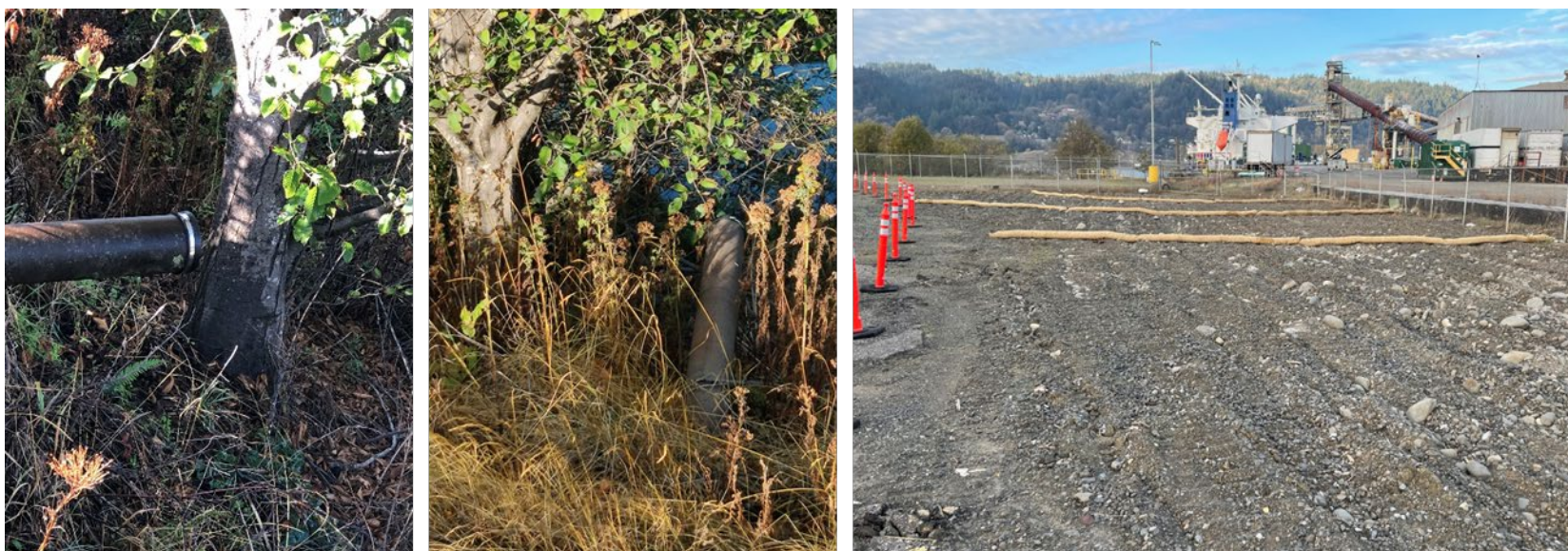
Figure 10. Basin K2 Stormwater SCMs (left: capped Basin K2 outfall; center: top view of capped Basin K2 outfall; right: scarified surface and wattles)
