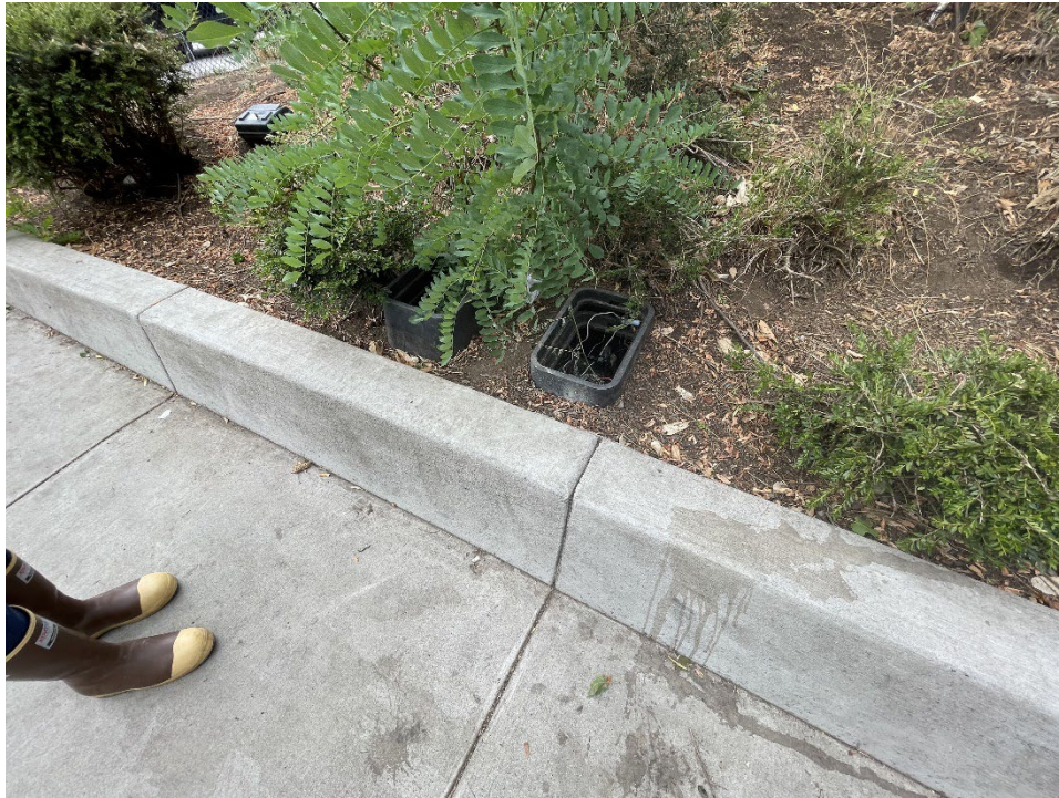
Photograph 19. Uncovered irrigation utility boxes.
