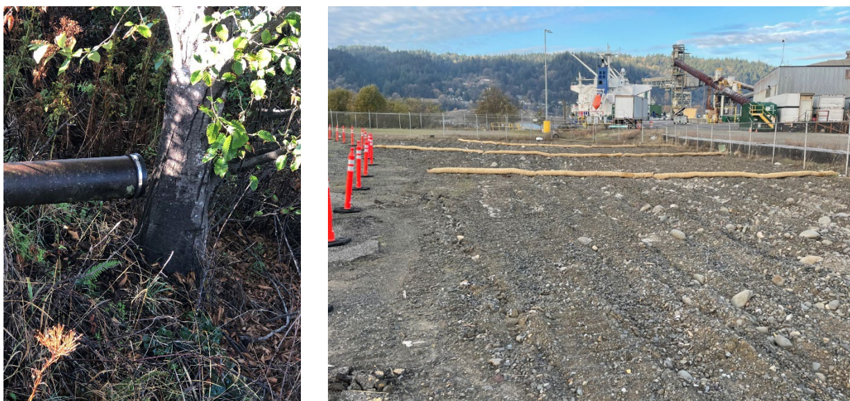
Figure 10. Basin K2 Stormwater SCMs (left: capped Basin K2 outfall; right: scarified surface and wattles)
