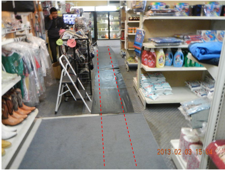
East leg after concrete pour – view north. Previous tenant.
