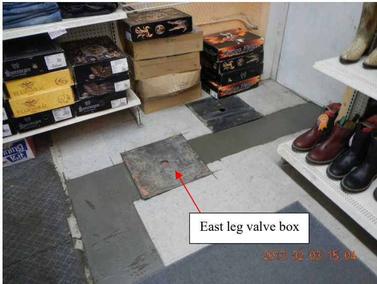
Collector line and valve boxes after pouring concrete – view southwest.
