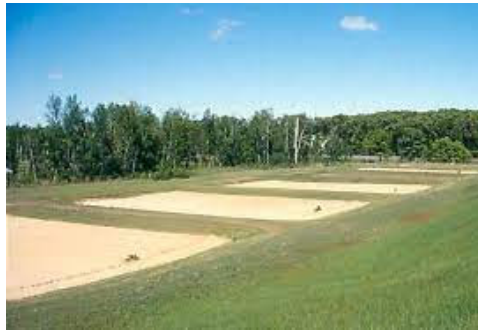
FIGURE 4-9: RAPID INFILTRATION BASINS
