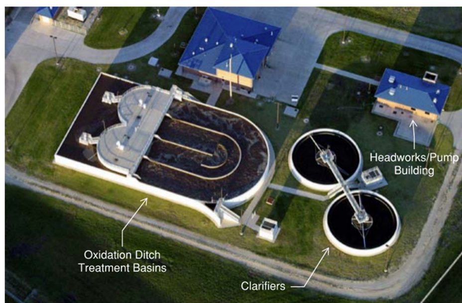
FIGURE 4-2: OXIDATION DITCH TREATMENT SYSTEM
