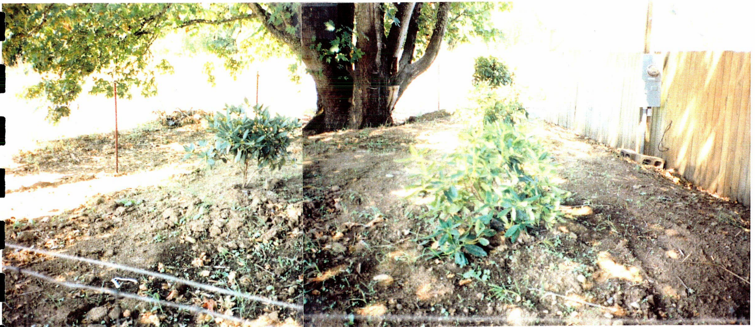
4. Close-up of soil disposal area. The aerated soil has been covered by 12 inches of clean fill.
