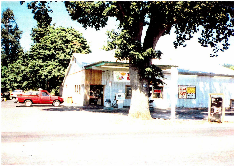
1. View of Meadowbrook Grocery from south, across South Highway 211.
