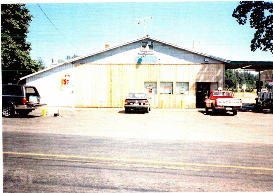
2. View of Meadowbrook Grocery from west, across Beaver Creek Road. Former tank locations marked by arrows.
