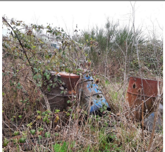
Photo 12: Outside used oil storage area near the AST: Containers being overgrown by blackberry bushes without secondary containment, labels, and multiple containers in poor condition.
