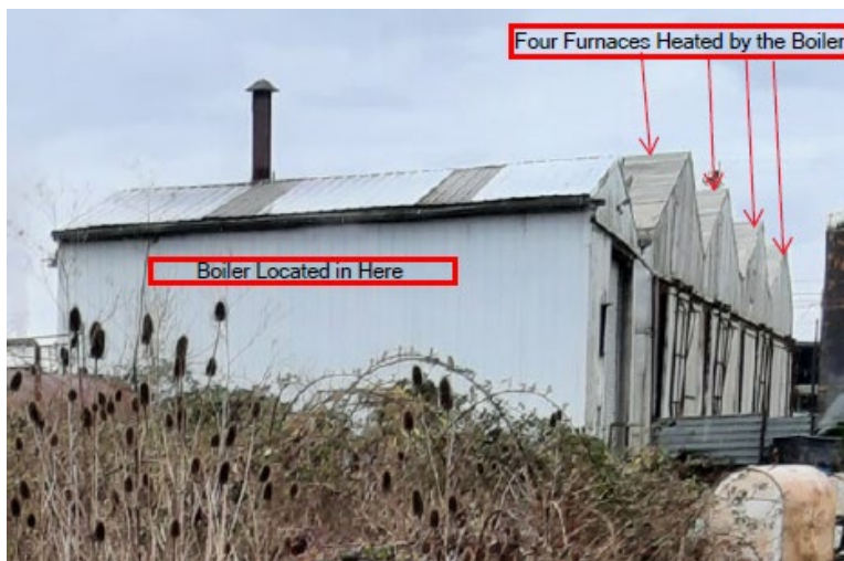
Photo 2: Building adjacent to the AST: The boiler (which can burn oil and natural gas) and four furnaces are housed in this building of five rooms.
