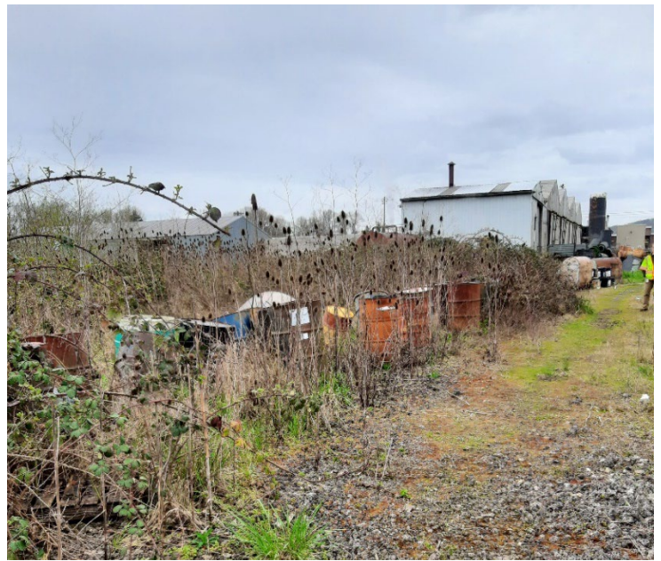
Photo 10: Outside used oil storage area near the AST ( The outbuilding in the background contains the boiler and furnaces ): Containers without secondary containment, labels, and multiple containers in poor condition. The containers were observed to contain contents.
