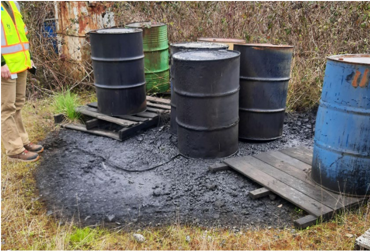
Photo 5: Outside used oil storage area near the AST: Close-up of containers without secondary containment, labels, and used oil leaking onto the ground. This is the largest spill area. The containers were observed to contain contents.
