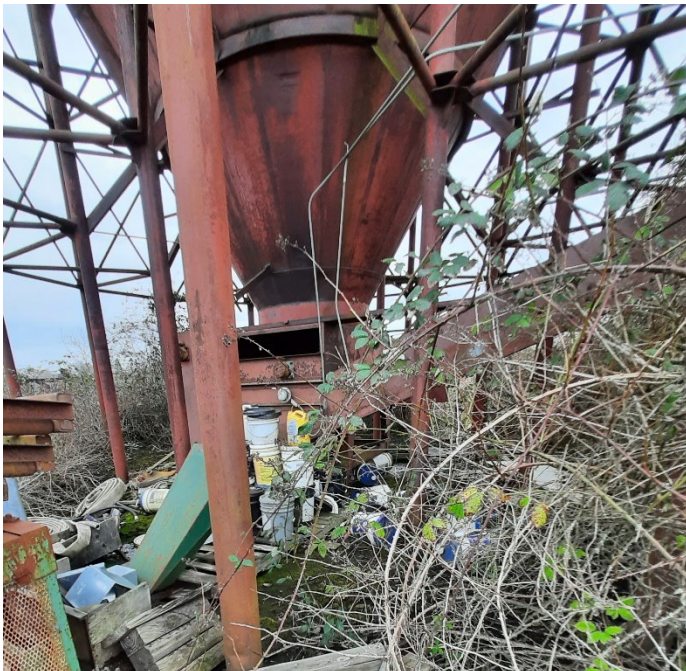
Photo 23: North road of facility: Multiple chemical containers being stored outside without secondary containment. The containers were observed to contain contents.
