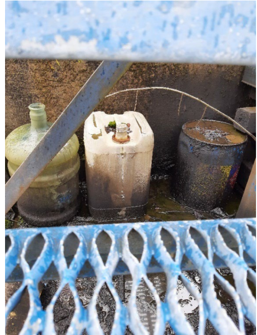
Photo 14: Outside under the steps that lead to the AST secondary containment: Containers in poor condition with what appears to be oil splatter coating them and the ground. Photo taken: April 21, 2023
