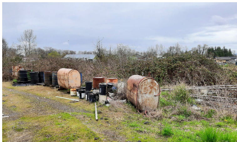
Photo 3: Outside used oil storage area near the AST: Containers without secondary containment, labels, and multiple containers without lids. The containers were observed to contain contents.
