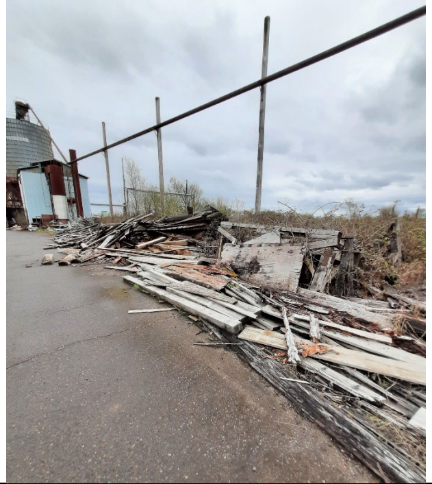
Photo 22: North road of facility: What appears to be waste materials being stored on the side of the road.
