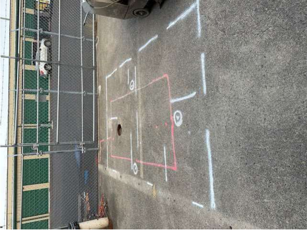
View of the marking identifying buried waste oil tank.
