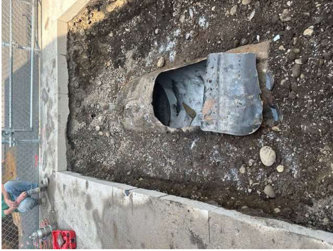
View of the 550 gallon waste oil tank, cut open and cleaned.
