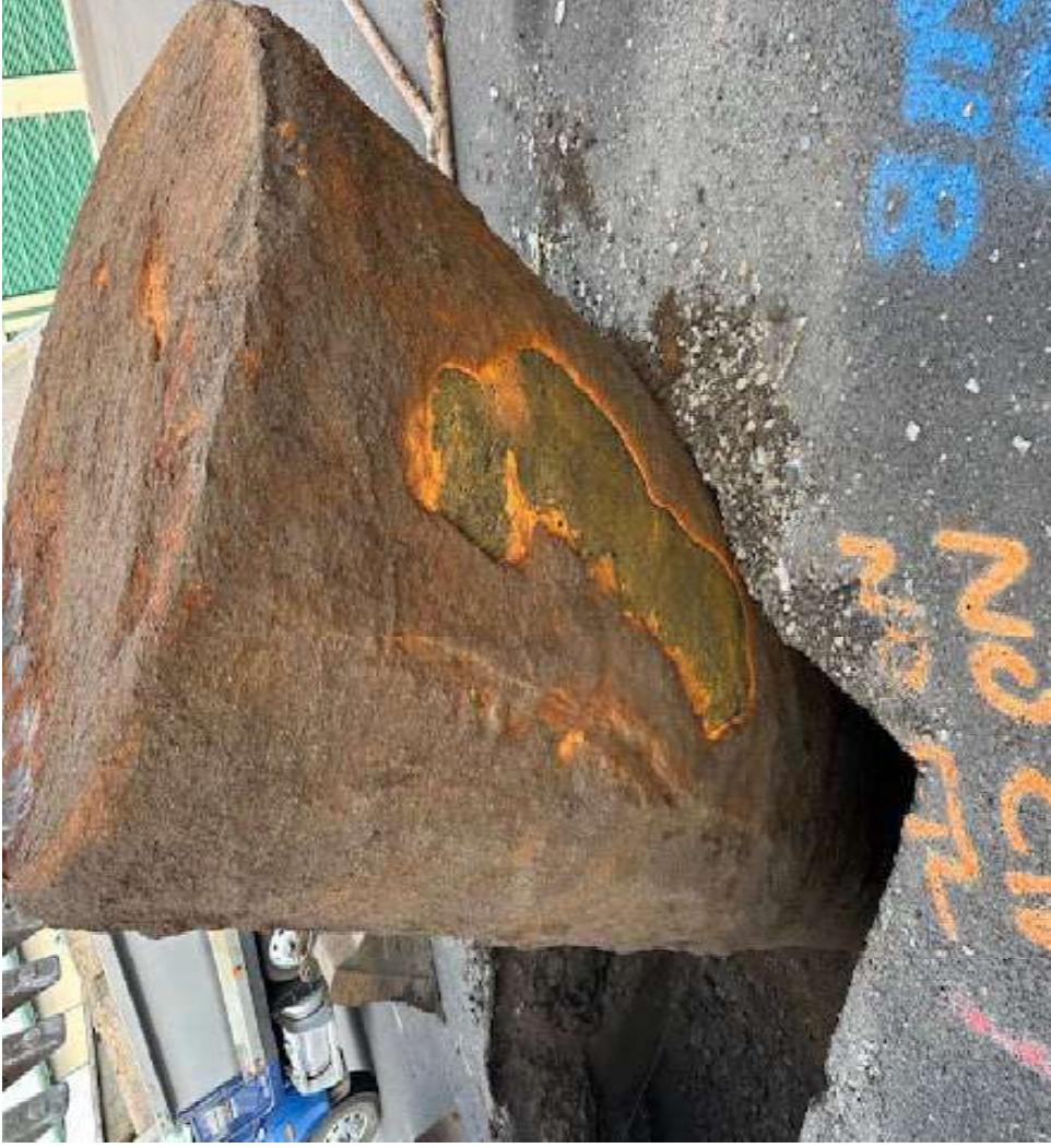
View of the base of the 1000 gallon gasoline tank.
