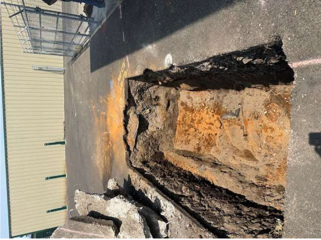
View of the gasoline tank excavation after removal/
