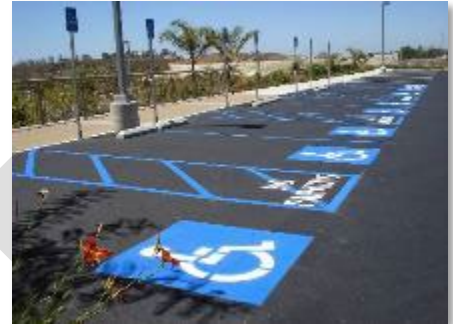
Example: ADA compliant striping (surface lot)
