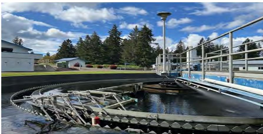
Secondary Clarifier brushes replaced to reduce the accumulation of algae along the weirs.
