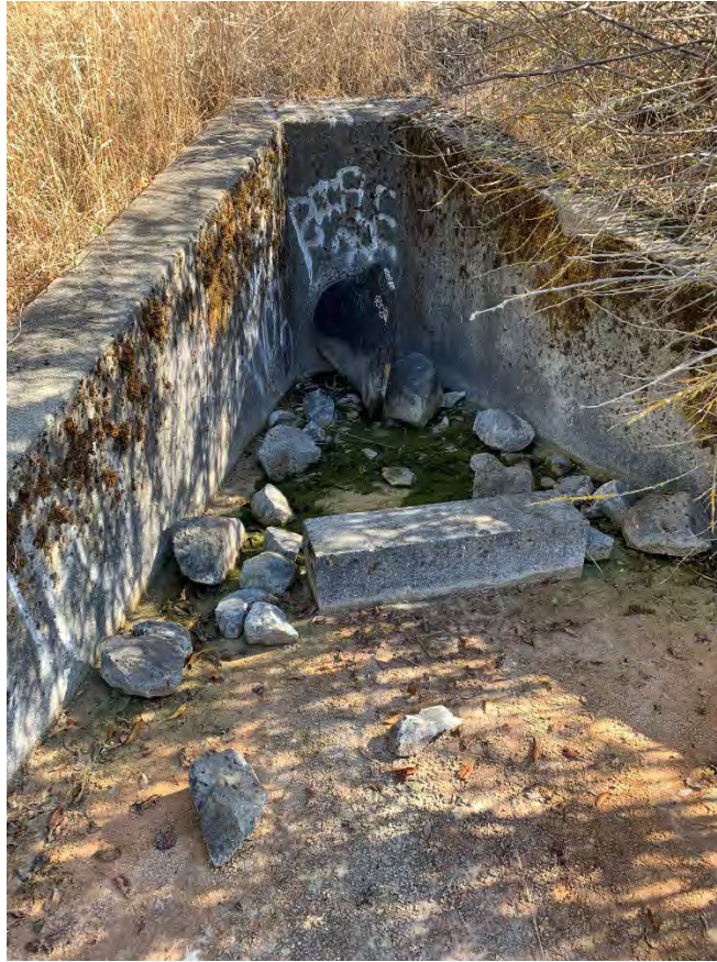
Photograph 3: Stormwater outfall was dry during inspection. View facing east.
