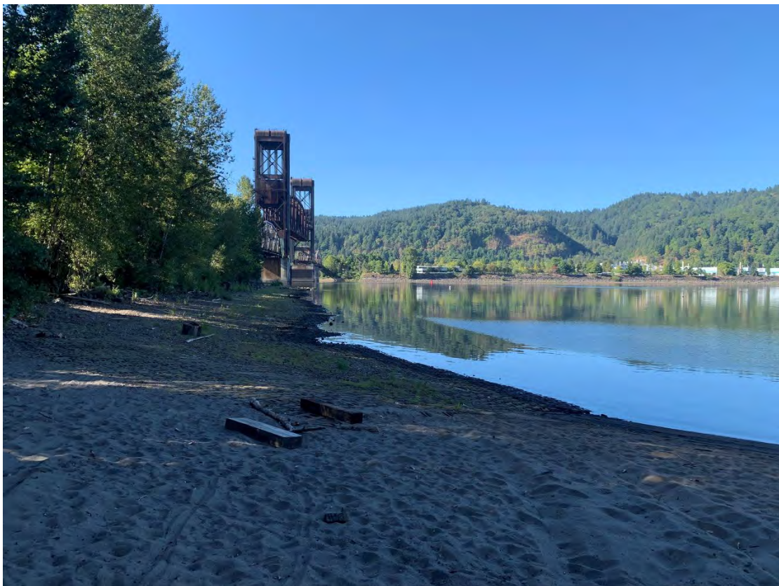
Photograph 1: Willamette Cove shoreline conditions. View facing west.
