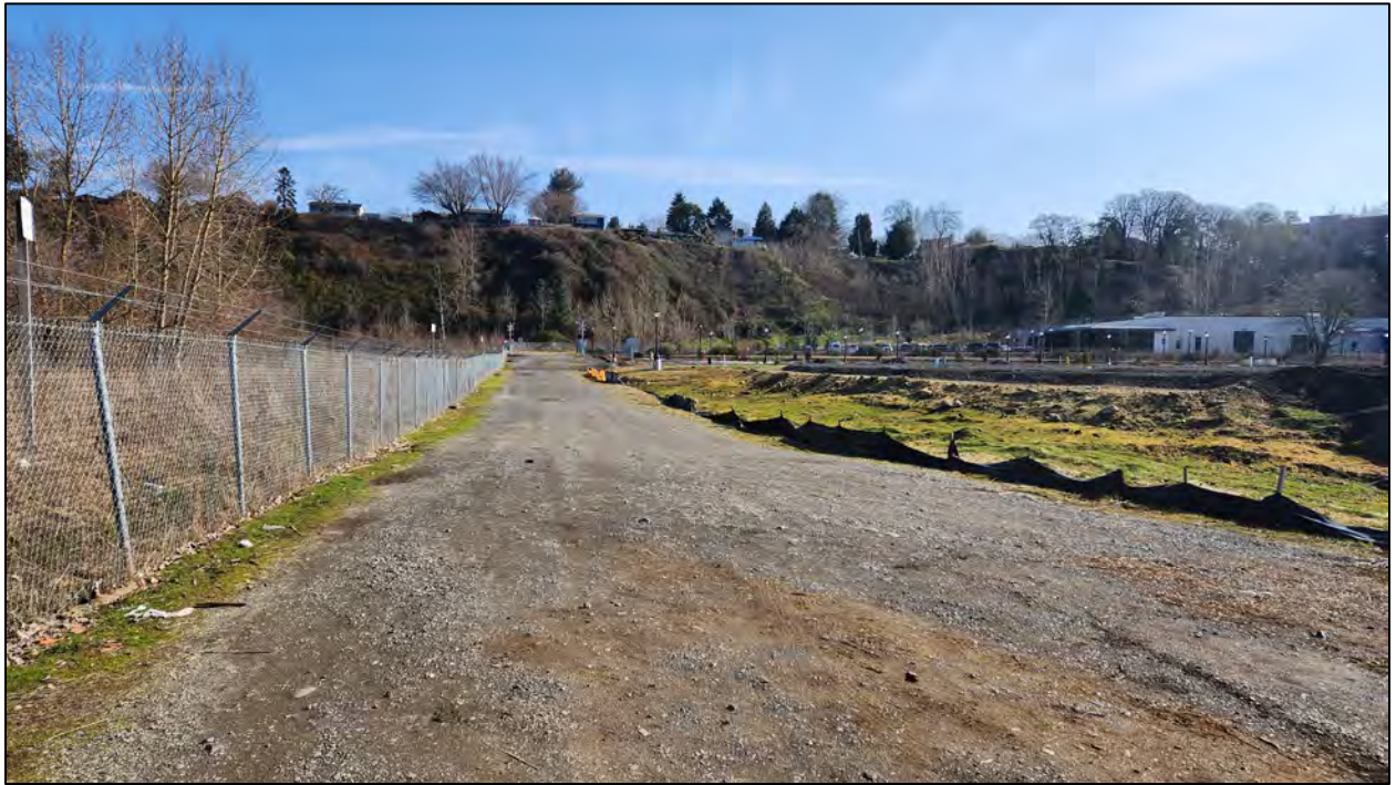
Photograph 6: Western end of N. Van Houten Place that will be raised approximately 3 feet during upcoming University of Portland improvements to the road. View facing east.
