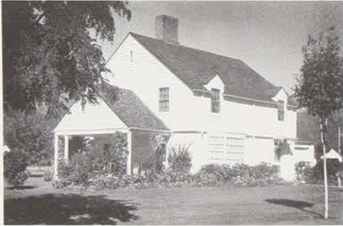
One of twenty frame houses for permanent staff.
