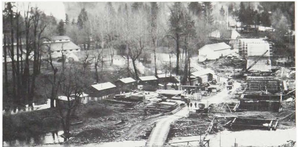
Bonneville hatchery grounds during construction of Tanner Creek Viaduct.
