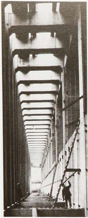
Dewatered fish collection channel at first powerhouse.
