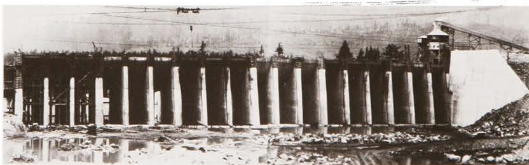
Upstream side of powerhouse substructure showing intake piers.
