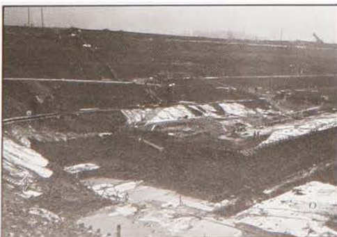
Placing concrete foundation for 2nd powerhouse.
