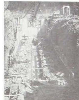
Excavation for main culvert and laterals in lock floor.
