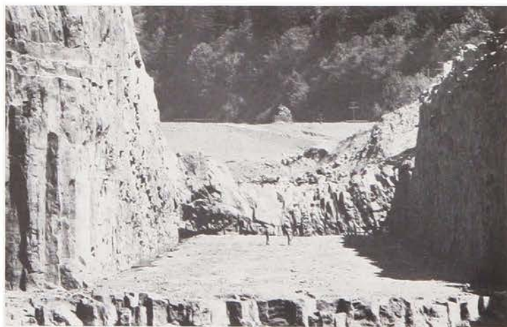
Excavation and rock trimming for lock and gate sill completed.
