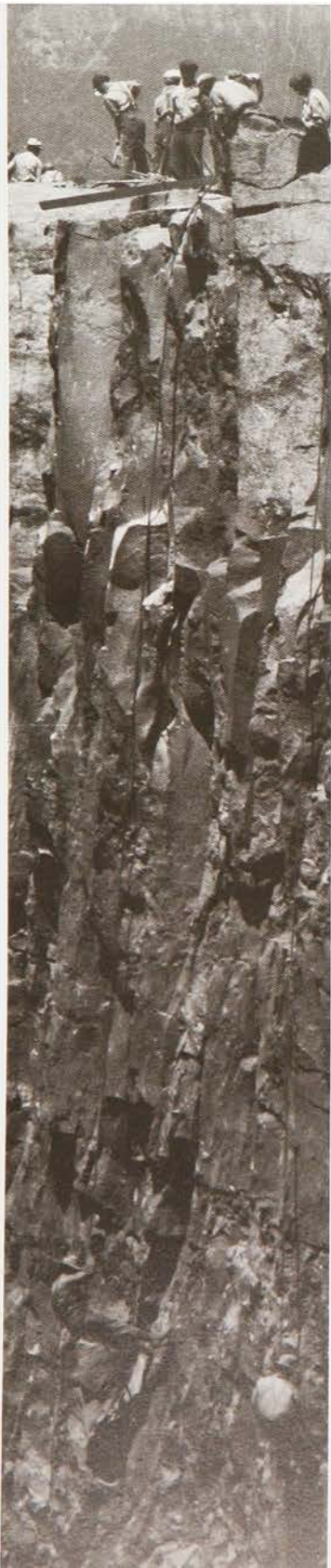
Workers scalping overburden and scaling down wall of lock.
