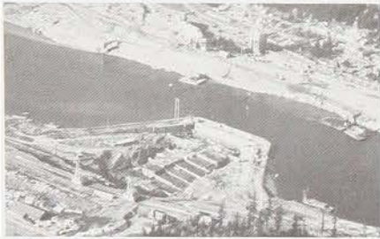
First step cofferdam completed.
