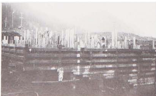
Crib 13 under construction. Note irregularities of bottom.
