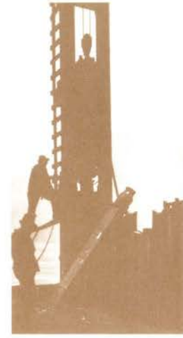
Pile driving sheet steel cofferdam face.
