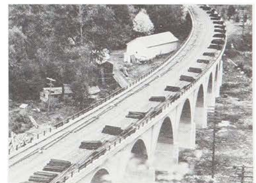
Tanner Creek railroad viaduct, awaiting installation of tracks.
