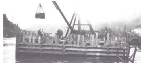
Crib in position. Pockets being filled.
