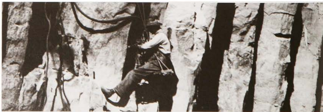
Workers scalping overburden and scaling down wall of lock.
