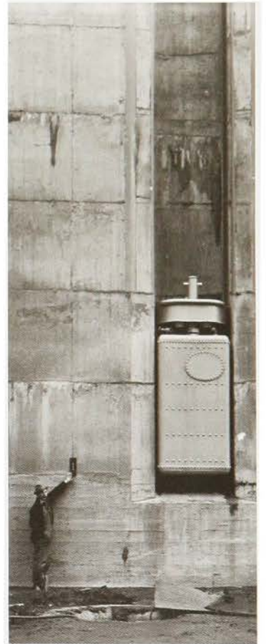
Floating mooring bit installed in lock sidewall.
