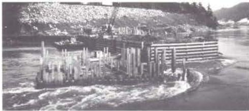
Crib towed into position for 2nd step cofferdam.
