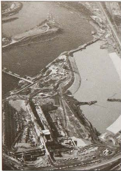
Second powerhouse under construction within cofferdam.
