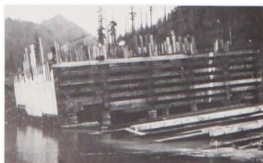
Crib on skids ready to be launched.
