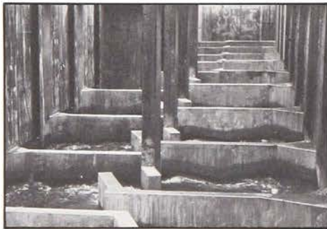
Vertical slot exit control section.
