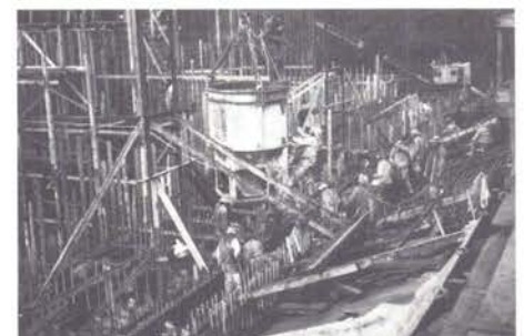
Pouring concrete in powerhouse substructure.
