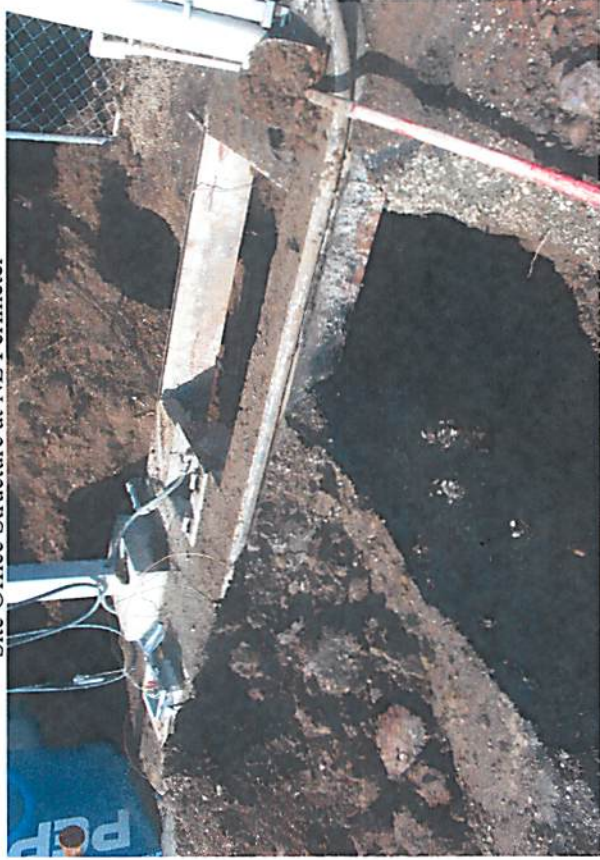
East Diesel Dispenser and Piping Trench Area
