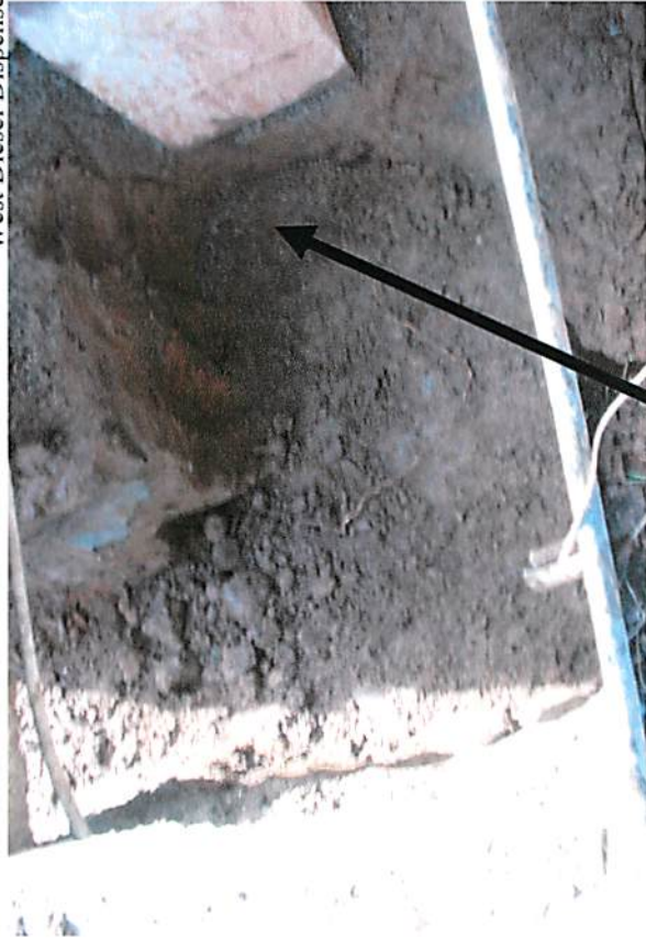
PCE Remains at Base of Canopy Footing
