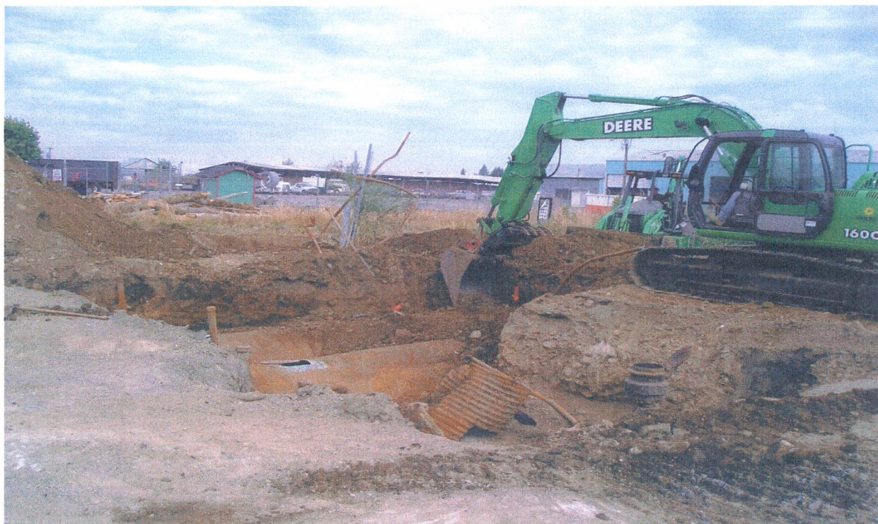
Excavating to Tops of The USTs
