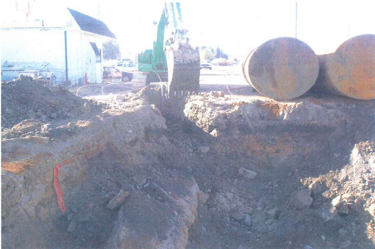
Bottom of UST Cavity (East Side) and Product Piping Trench
