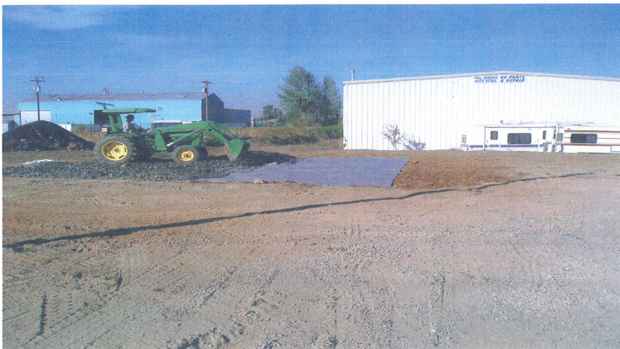
Backfilled UST Cavity with Contaminated Soil Stockpile in Left Rear.
