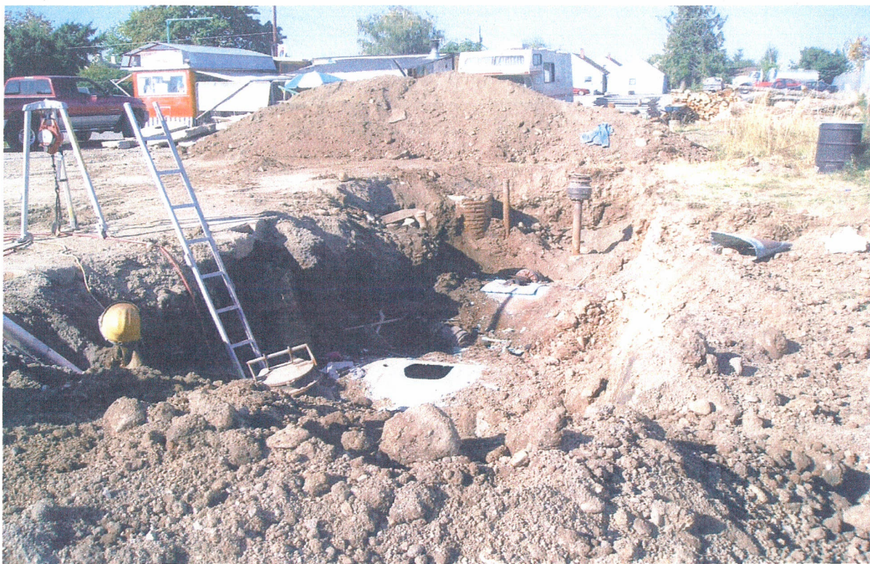
Fill Ends of USTs Exposed
