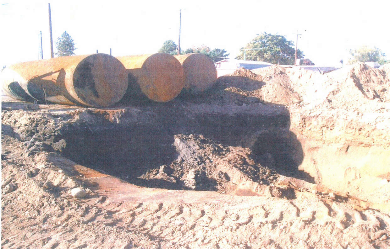
Three of the Four USTs Awaiting Transport
