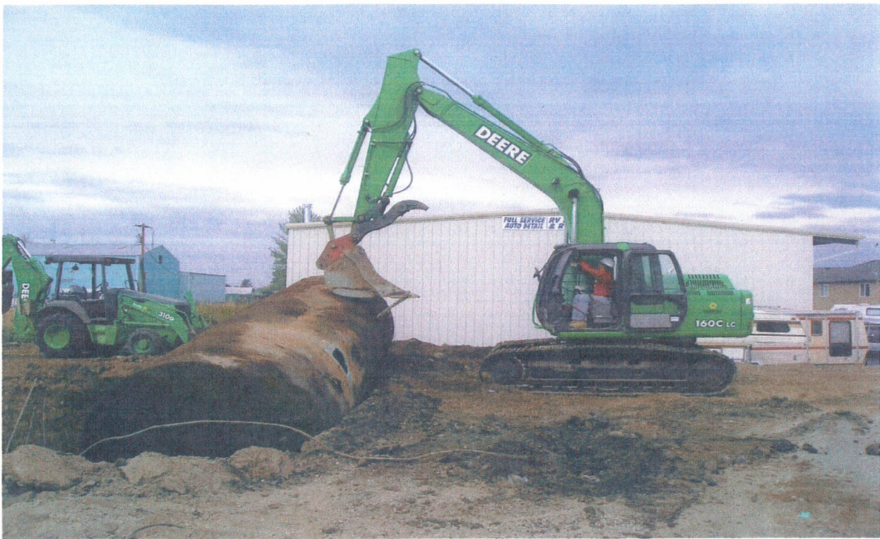
Removing Tank No. 1 (Eastern UST)
