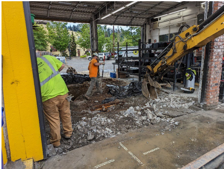
Expanding the limits of excavation EX01 on June 20, 2023.
