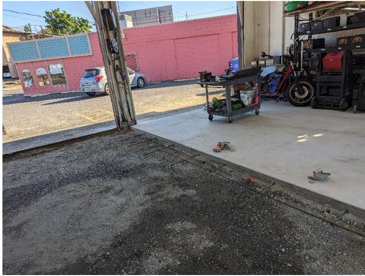
Backfilled and compacted excavation EX01 view south.
