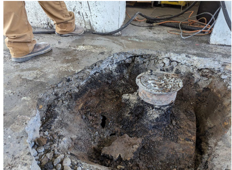
Top of UST01 exposed on June 19, 2023.
