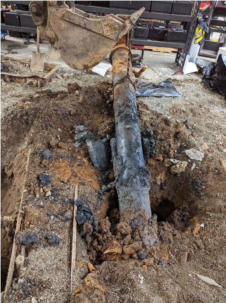
Hoist H01 on ground after being removed.
