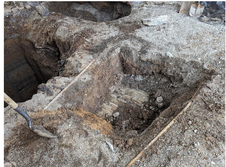
View of excavation EX02 where SUMP01 had been located.
