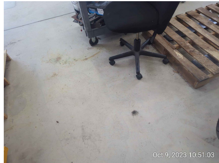
Post sample photo showing floor slab patched with hydraulic cement.
