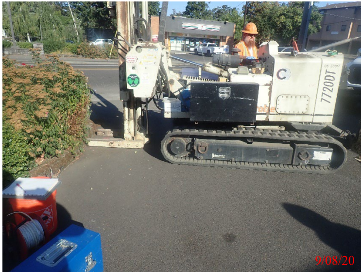
Using a drill rig to drill boring EB04 near former gasoline UST pit.
