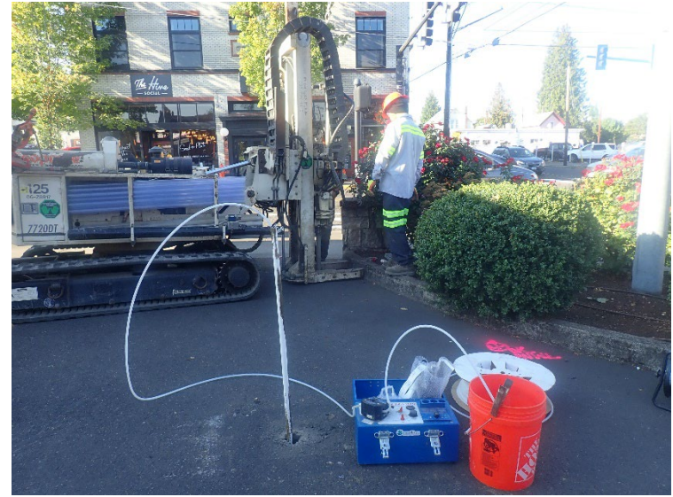
Collecting reconnaissance ground water sample from EB04, view south.
