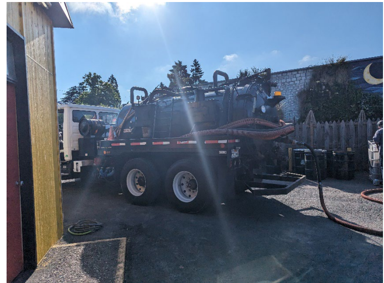
Tide Water pumping the liquid contents of tote from the used oil UST and drums of used oil from the hoists into a tanker truck for disposal.
