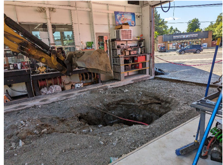
Limits of excavation EX03 in West Service Bay.
