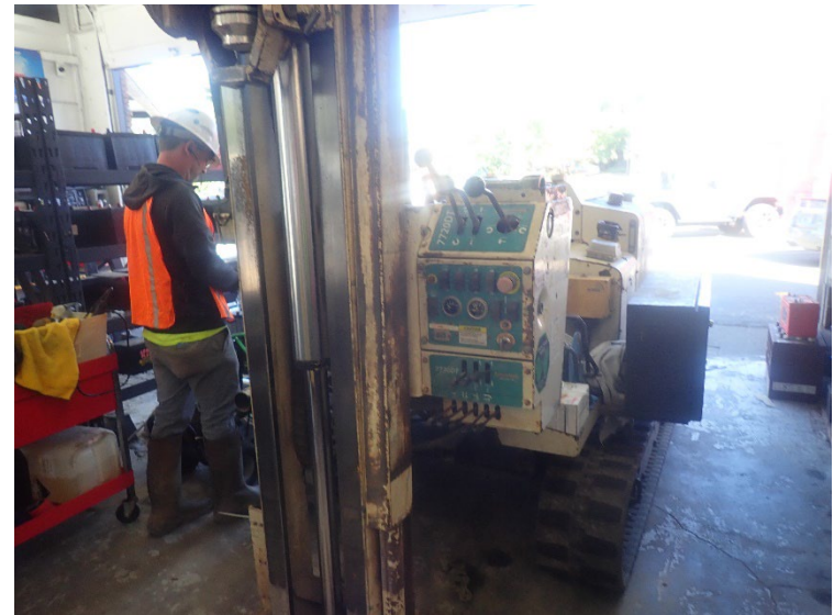
Drill rig advancing EB03 inside building next to UST01.
