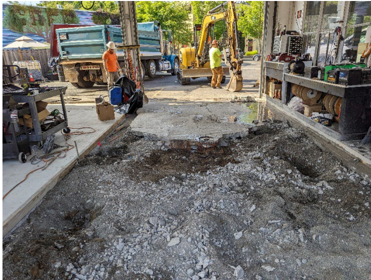
Exposing hoist H03.
