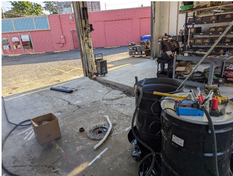
Hoist H03 in West Service Bay.
