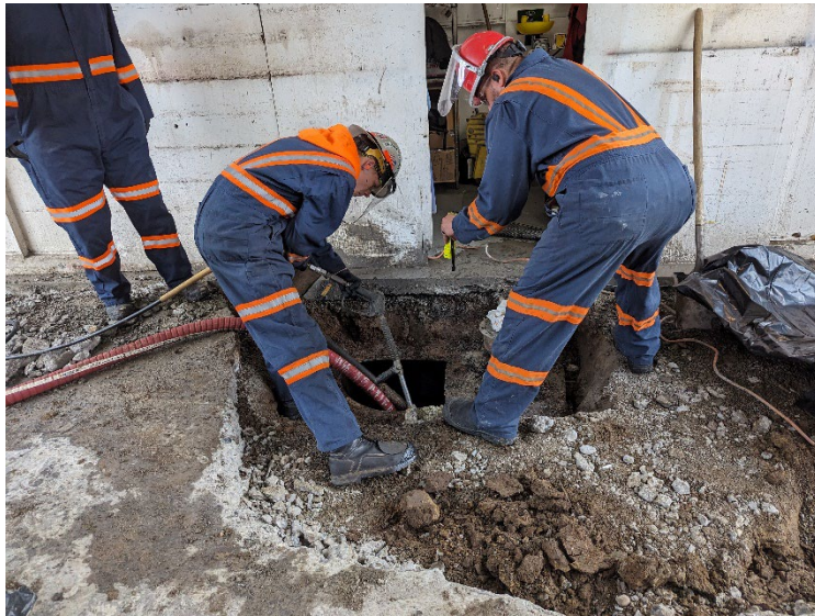
The interior of UST01 being thoroughly cleaned.
