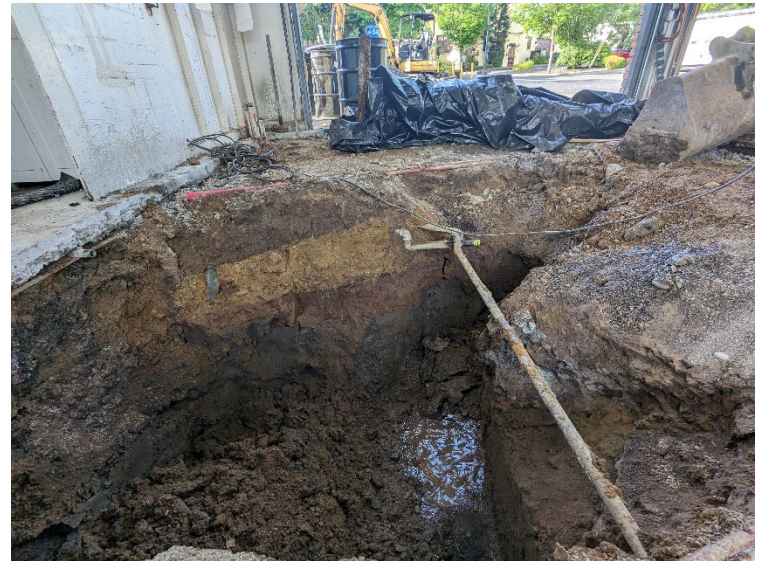
View of EX01 on June 20, 2023. Note band of stained soil (PCS) in sidewall.
