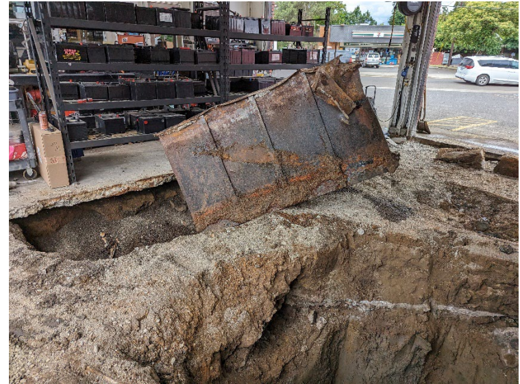
Removing unknown sump feature (SUMP01) from East Service Bay.
