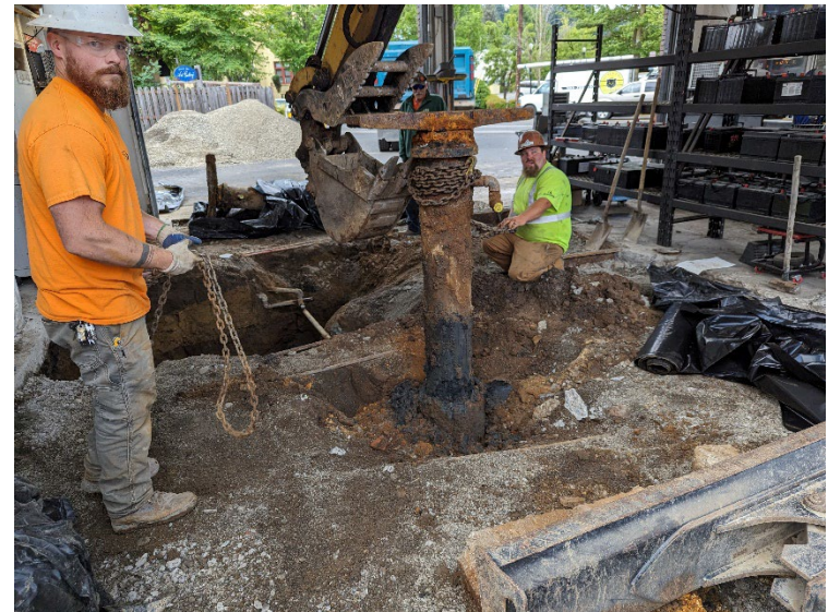
Pulling hoist H01 from the ground.
