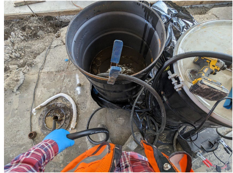
Pumping oil contents from hoist H03 into a drum.
