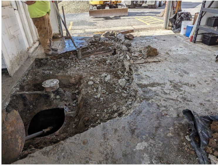
View south at UST01 after cutting a hole in its top. Note vent pipe heading east.
