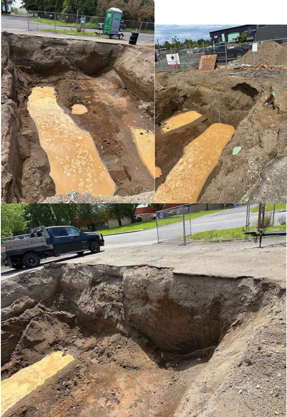
View looking south. The diesel tank is to the right and gas tank to the left. No soil contamination was observed at the south ends of the tank.
