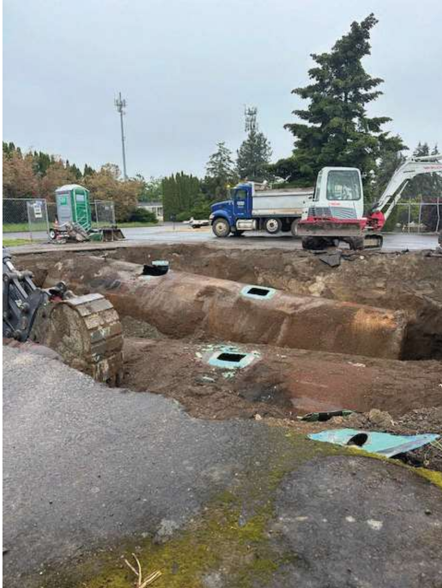
The tanks were lifted and pulled away from the original positions, to ease lifting out of the ground, and loading unto haul away truck.
