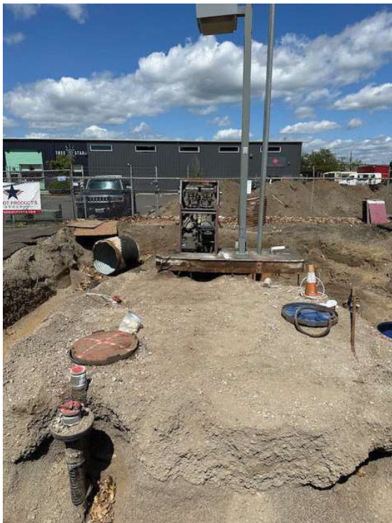
Pictures of the concrete pad removal above the tanks on May 7, 2024. The concrete was taken to disposal site as fill. The concrete did rebar.
