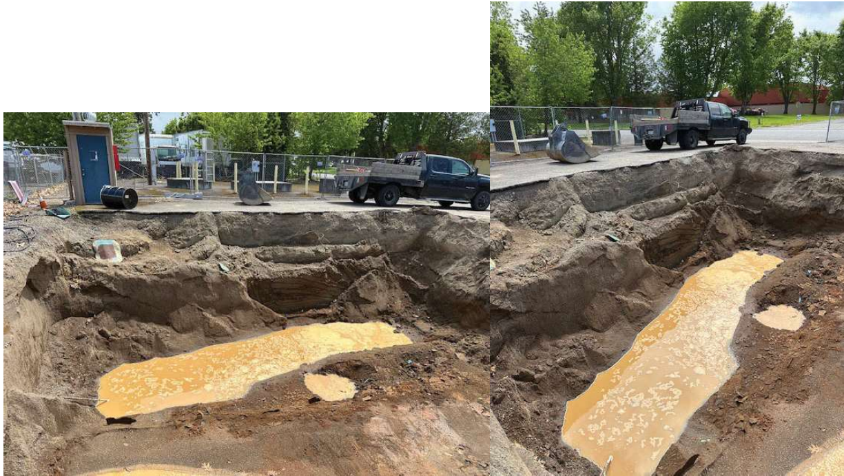
Views of the gas tank pit after removal of the gas tank. Soil samples were collected at each end of the gas tank. The circle hole is where a soil samples were collected between the tanks.
