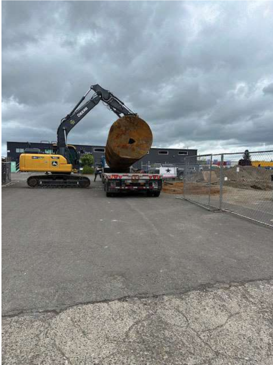
View of diesel tank being loaded onto a truck for recycling on May 22, 2024.
