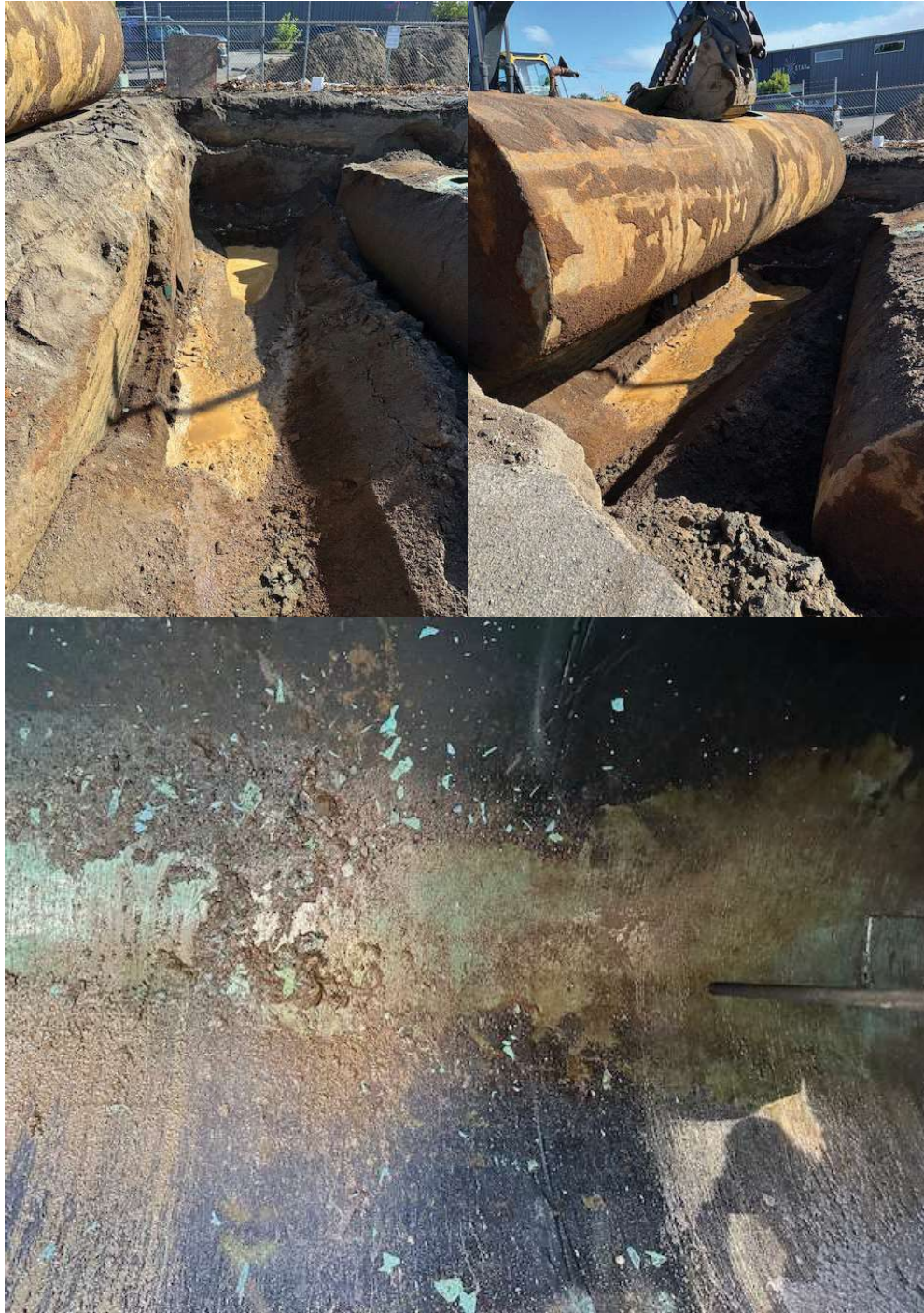
Views of the diesel tank lifted from the ground. Groundwater was observed under the tank at a depth of 11.5 ft. The diesel tank had no observable holes from corrosion. The interior of the diesel tank showed no observable pits or holes. There was a dusting of dirt inside of the tank.
