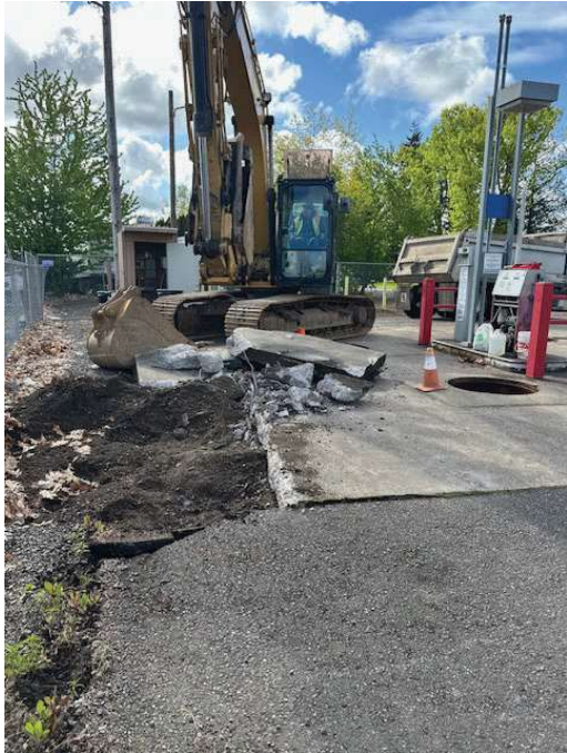
Pictures of the concrete pad removal above the tanks on May 7, 2024. The concrete was taken to disposal site as fill. The concrete did rebar.
