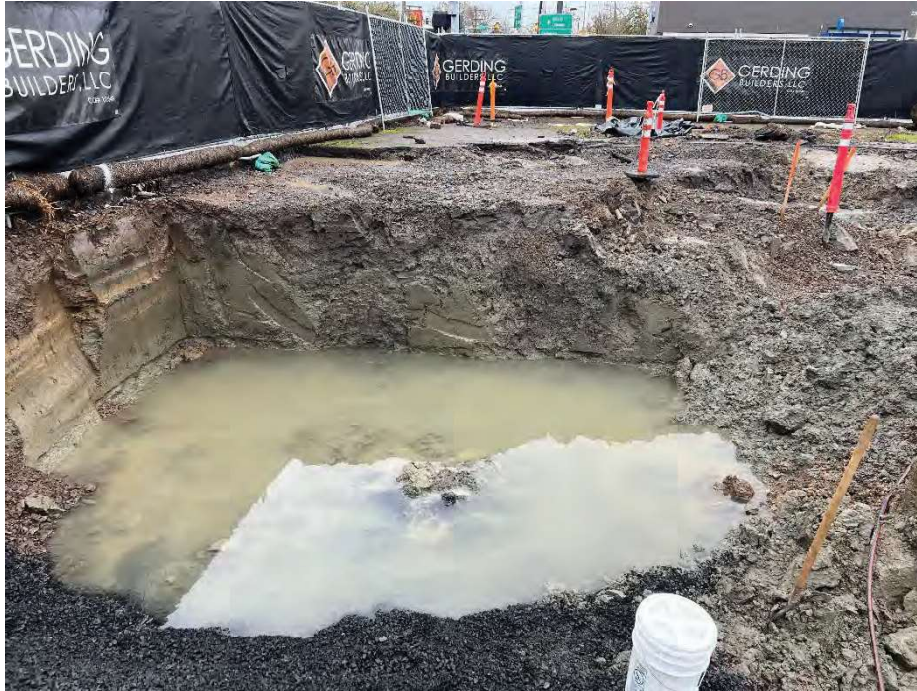
Photo 1. Looking east toward the at the former location of UST-01. Contaminated water spilled from the tank during removal and was subsequently pumped and containerized. The water visible in the photo is groundwater that recharged into the excavation following pumping.
