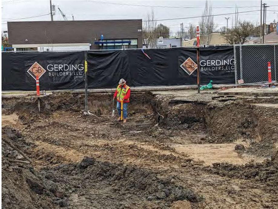
Photo 3. PBS contracted Alpha Locates of Gaston, Oregon to scan the remainder of the site for additional underground storage tanks (USTs).
