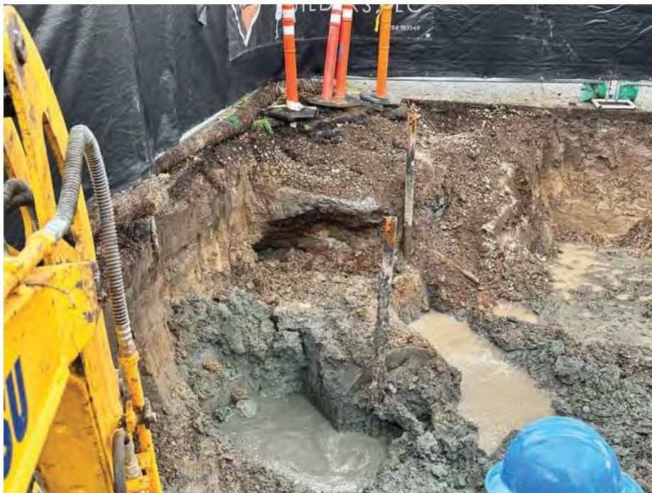
Photo 4. UST-02 was located near the northeastern corner of the site. It was observed to be previously decommissioned with controlled density fill (CDF).
