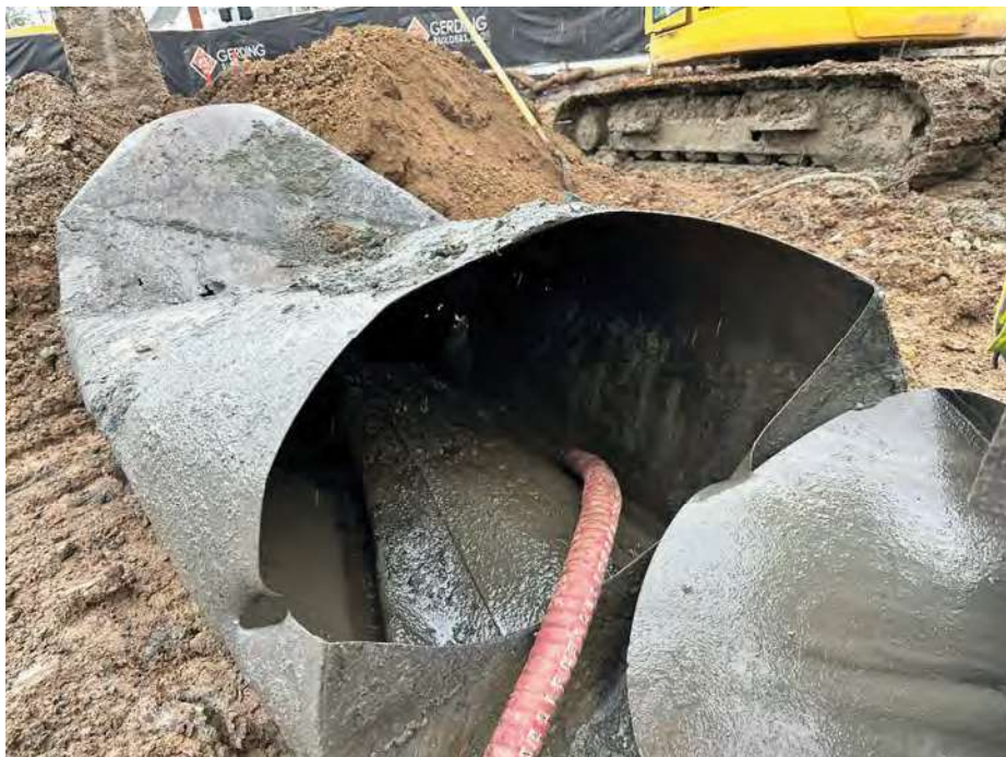
Photo 6. The tanks were cleaned with assistance from Cowlitz Clean Sweep (CCS) of Portland, Oregon. Following cleaning the tanks were disposed of at a recycling facility.
