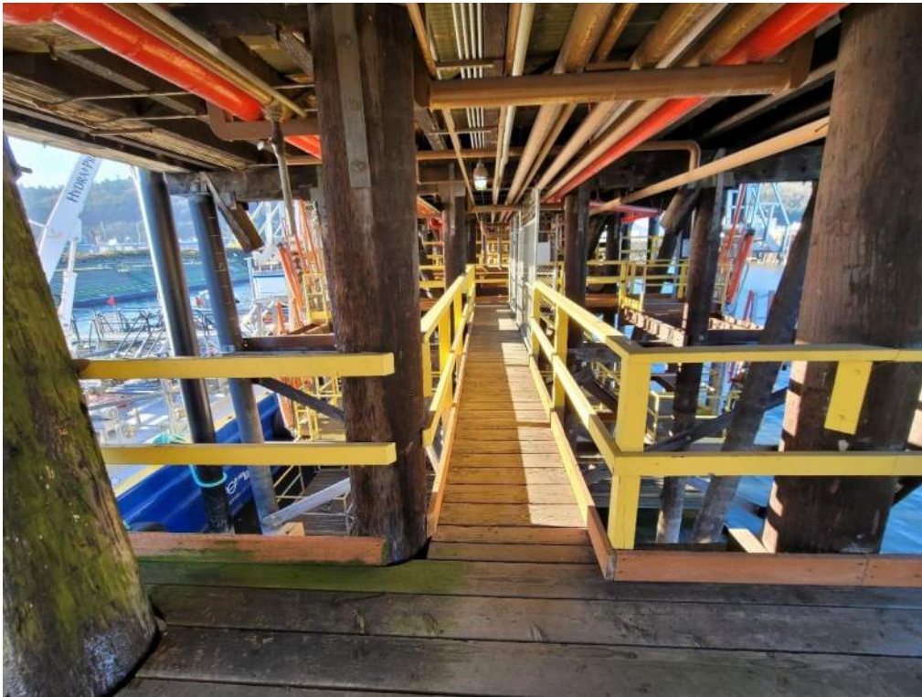
Picture 27. Substructure walkways and platforms.
