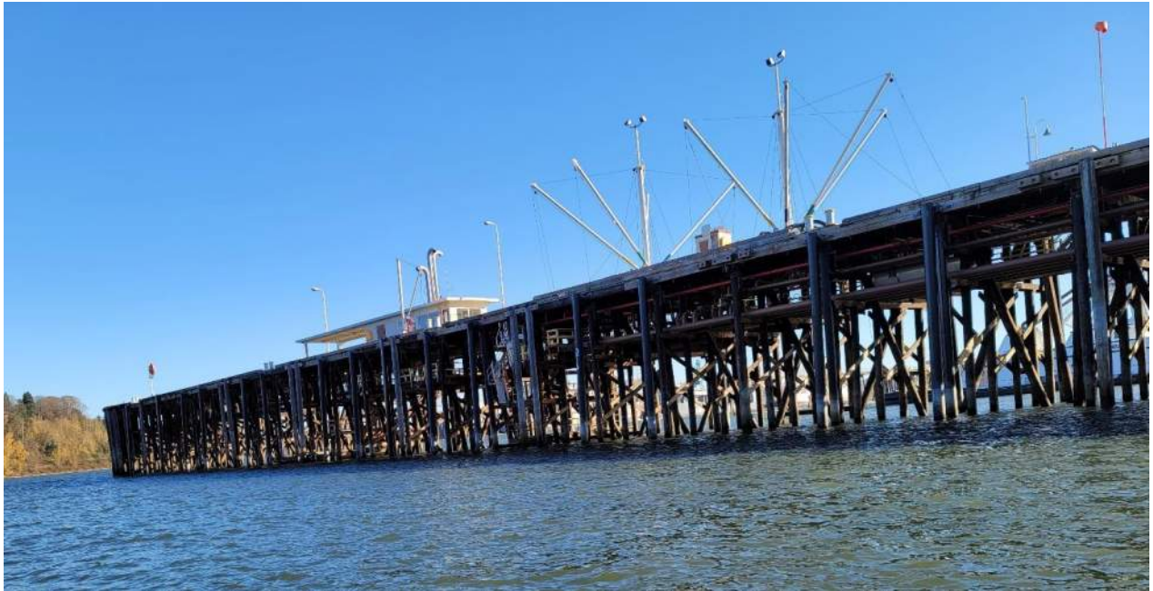
Picture 1. Downstream berth and service area.
