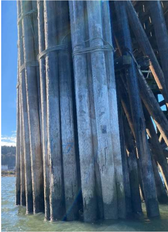
Pictures 11,12, 13, and 14. Pier head cluster piles. Note broken and missing piles, dead heads at either corner, broken and missing piles at head.
