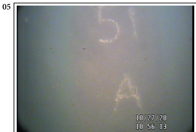
Pile 51 A - Loose at top.
