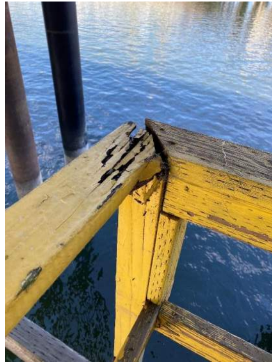
Pictures 35 and 36. Lower platform to floating deck in decay, Grid 46; handrail on third level broken at the corner connection.
