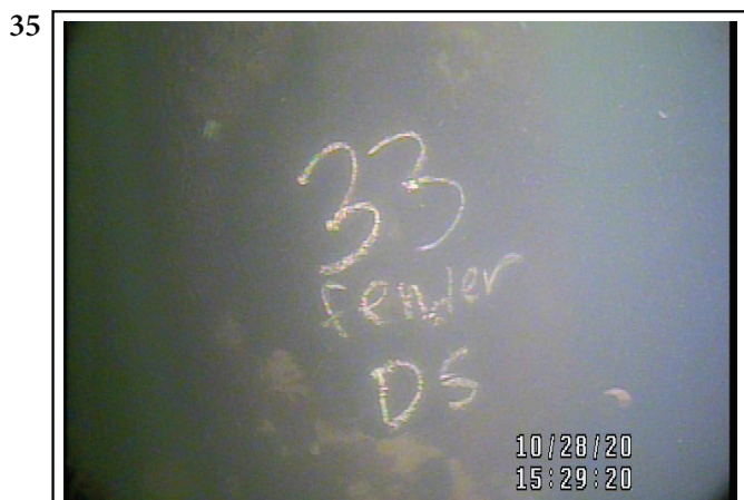
Fender Pile 33 Downstream side.
