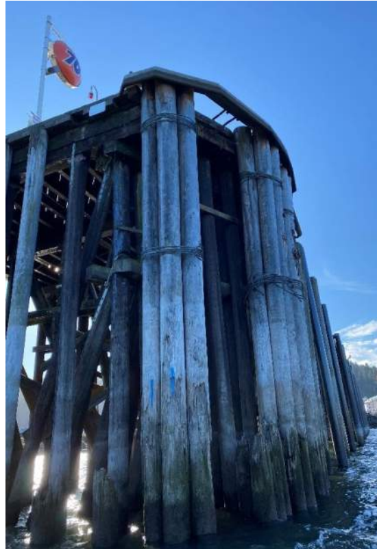
Pictures 11,12, 13, and 14. Pier head cluster piles. Note broken and missing piles, dead heads at either corner, broken and missing piles at head.
