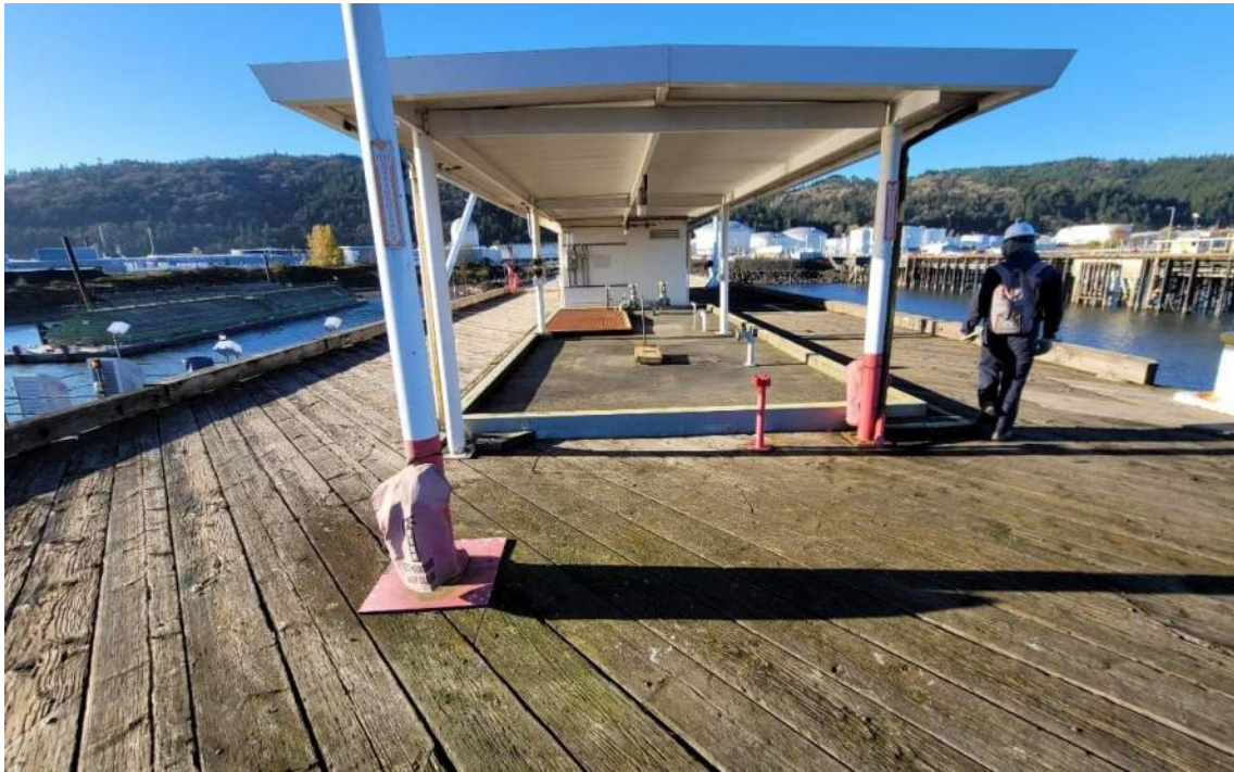
Pictures 23: Service area and secondary containment, riverside of the operations shack.
