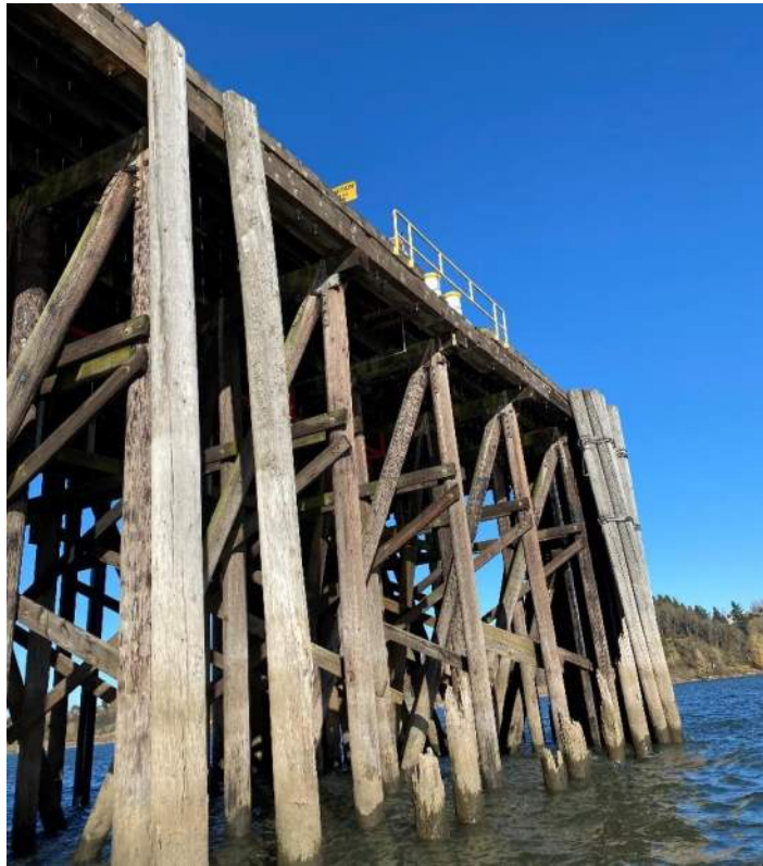
Pictures 15 and 16. Upstream berth, near head. Note broken/missing fender piles, exposed structure.
