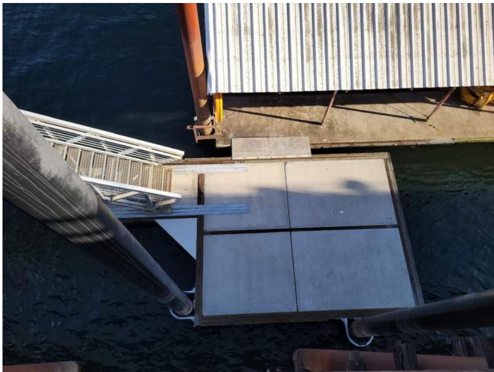
Picture 39. Boathouse, gangway landing, and guide piles (2021).
