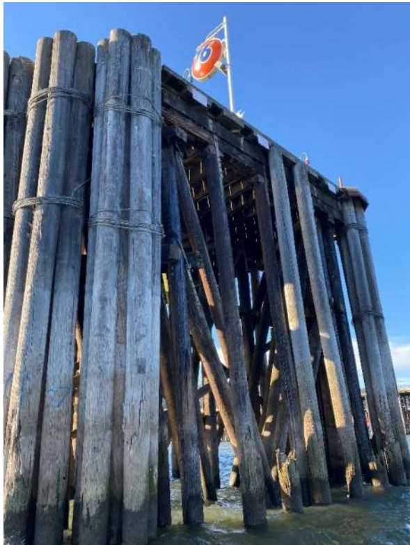
Pictures 11,12, 13, and 14. Pier head cluster piles. Note broken and missing piles, dead heads at either corner, broken and missing piles at head.
