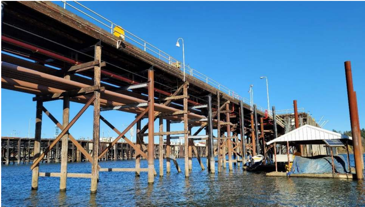
Picture 5. Pier approach and boathouse, upstream side.
