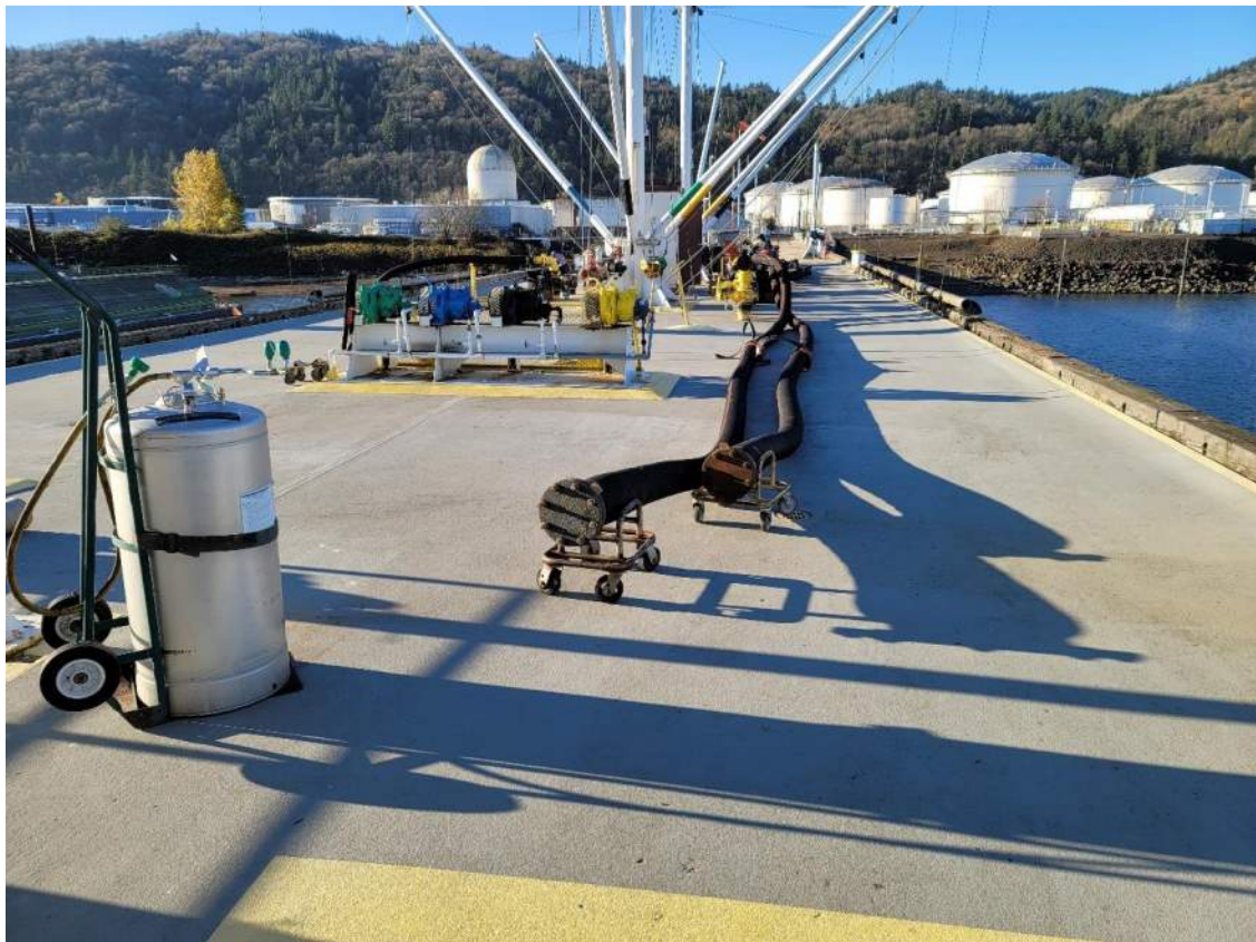
Picture 24. Service area. Note good condition of concrete surface.
