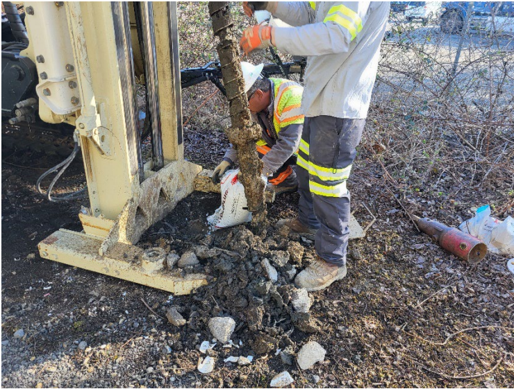
View of the sand pack and bentonite seal material caught on the auger flight while over drilling MW01.
