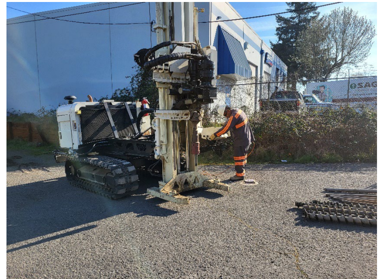
View of MW05 as the monument and casing / screen were removed.
