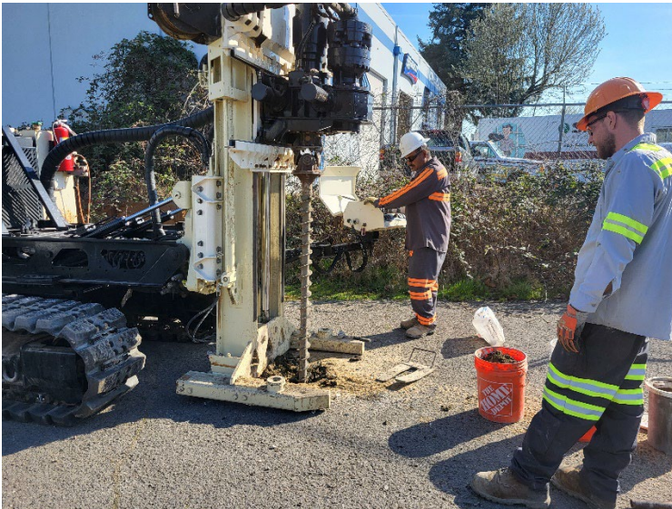
View of MW05 during over-drilling with auger tooling.
