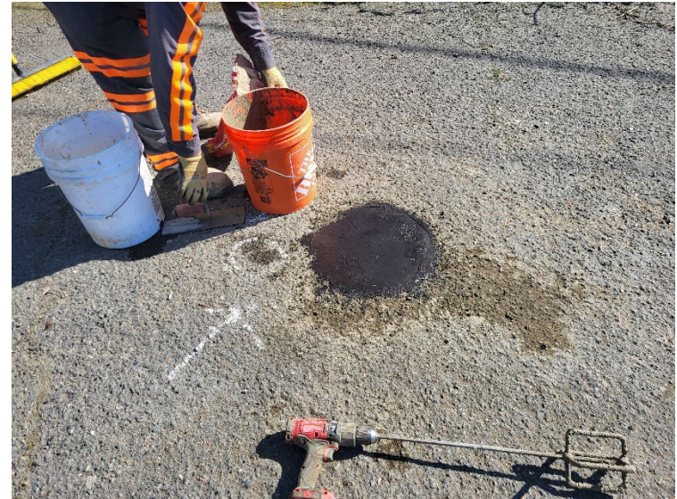
A concrete cap was installed over the bentonite chips at each well location.
