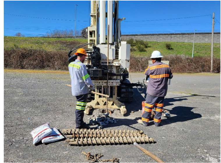
View of MW04 during over-drilling with auger tooling. Cuttings were contained in drums for appropriate disposal.
