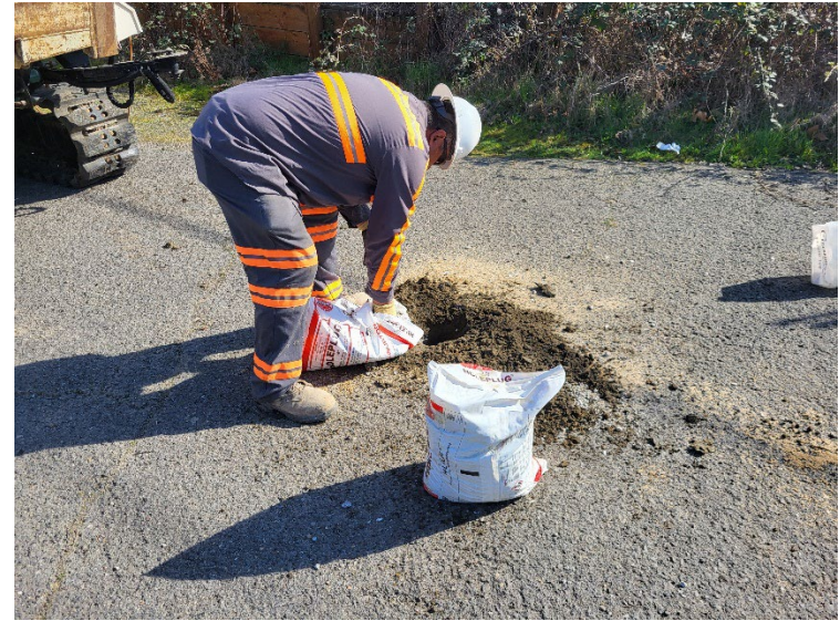
After over-drilling to total depth, all wells were abandoned using bentonite chips. View of MW05.
