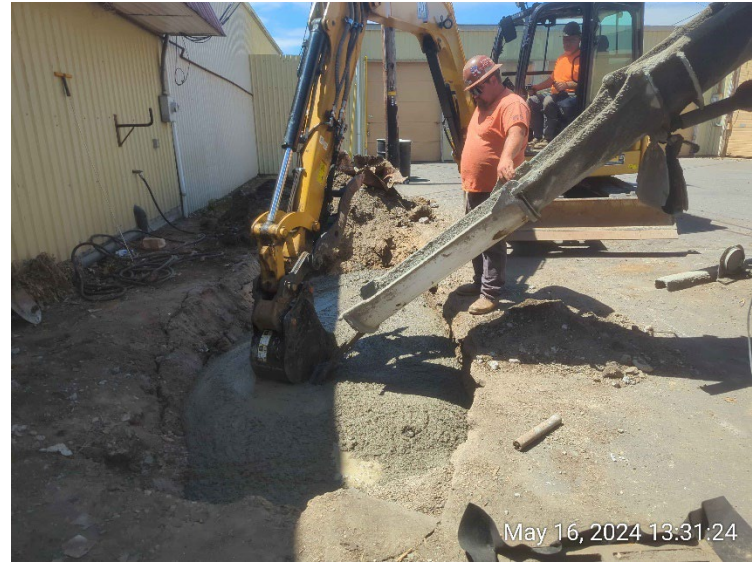
The CDF was allowed to completely fill and mushroom over the top of the septic tank to complete the decommissioning.
