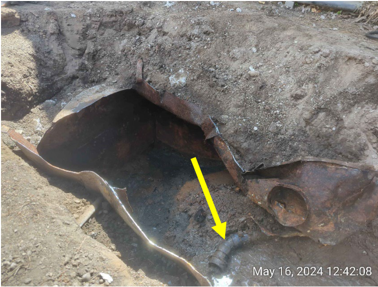
View of tank interior after pumping down the liquid contents revealing the former inlet pipe entering the south side of the tank (yellow arrow) and abundant sand.
