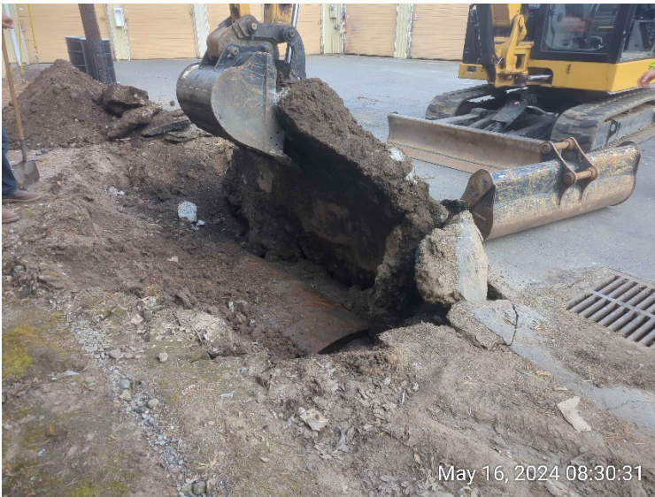
A concrete pad was found to overlay a metal tank structure. The concrete was broken up and hauled offsite for disposal.
