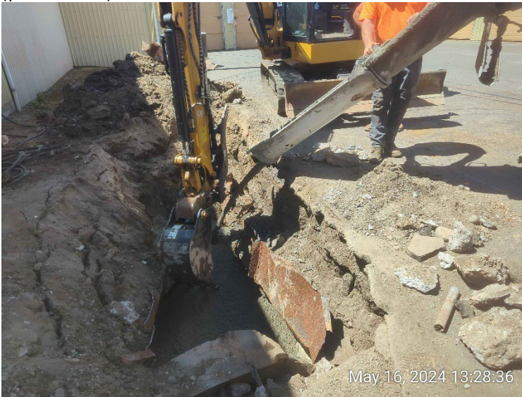
After an inspection from the City, authorization was granted to proceed with filling the tank with CDF.
