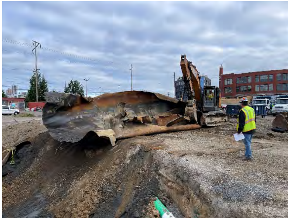
Photo #1 The former UST removed and opened.
