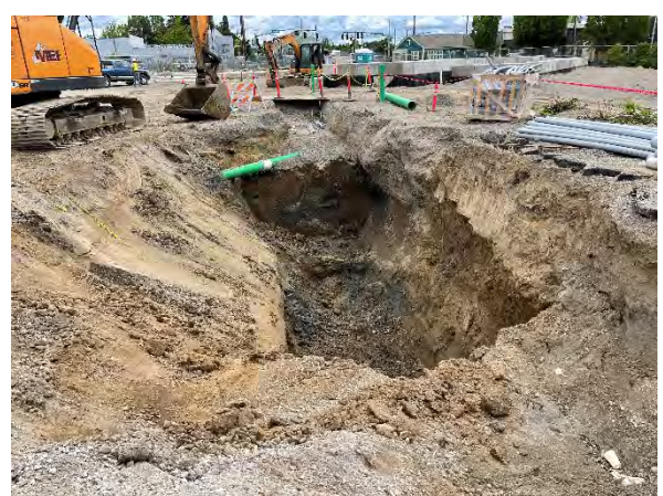
Photo #6 Post soil removal. Small residual soil contamination beneath active sewer line.
