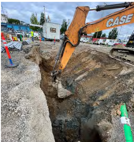
Photo #5 View of pit facing west while removing impacted soil
