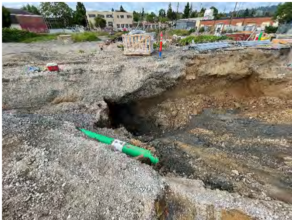
Photo #3 Exposed sewer line in east end of pit.
